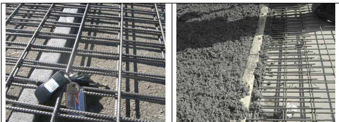
Figure 34: Placing construction joint: sponge underneath of mesh.
