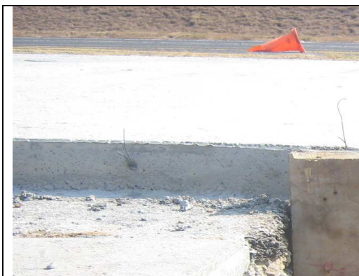
Figure 28: First side of type 1 longitudinal joint
