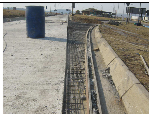
Figure 2: Metallic lipped channel side-forms of UTCRCP
