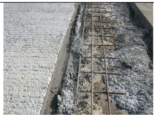
Figure 29: First side of type 2 longitudinal joint
