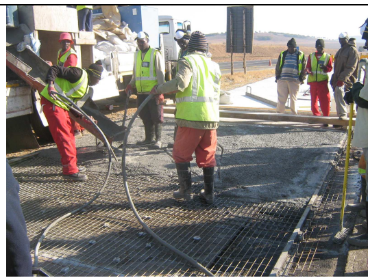
Figure 21: Concrete vibration using pocket vibrator
