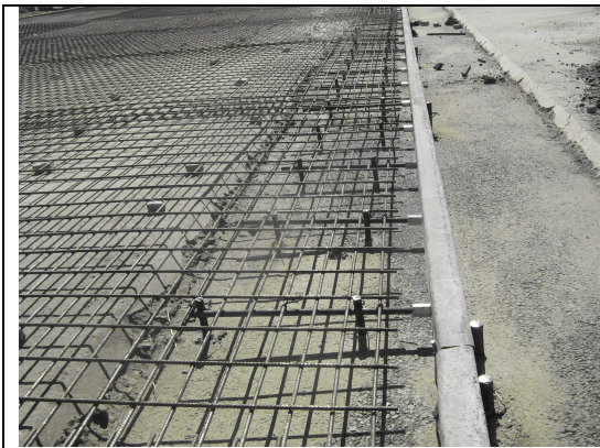
Figure 10: form-work of joint using tie bars with Hex coupling nut (Type 1)
