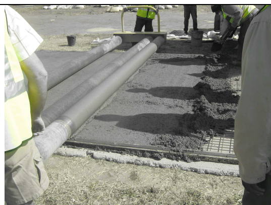
Figure 23: Oscillating triple roller screed in action
