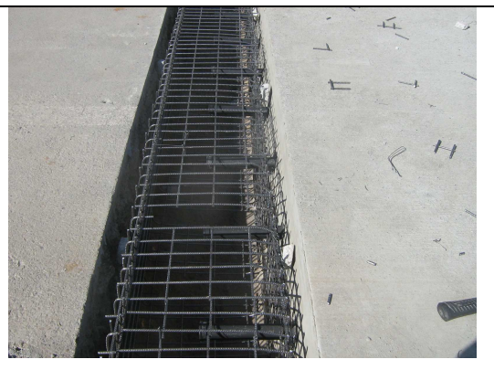
Figure 13: Reinforcement for anchor beam
