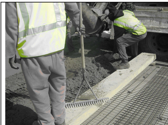
Figure 20: Pouring and spraying of fresh concrete
