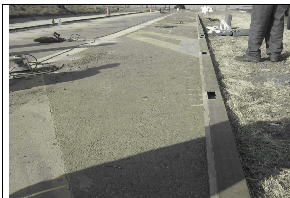
Figure 1: Rectangular metallic tube side-forms of UTCRCP
