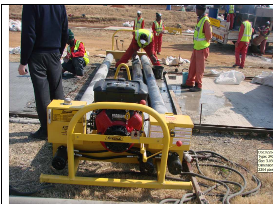
Figure 22: Oscillating triple roller screed
