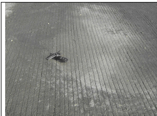
Figure 38: Tinning surface finishing.
