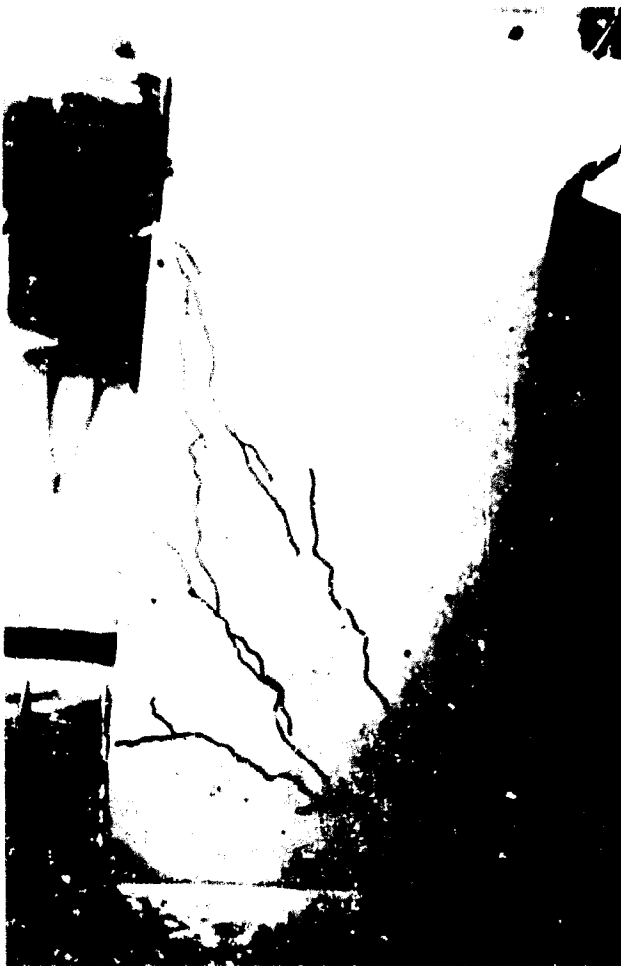
Figure B.30: Crack pattern of Column 1C seen from one side after the impact phase.
