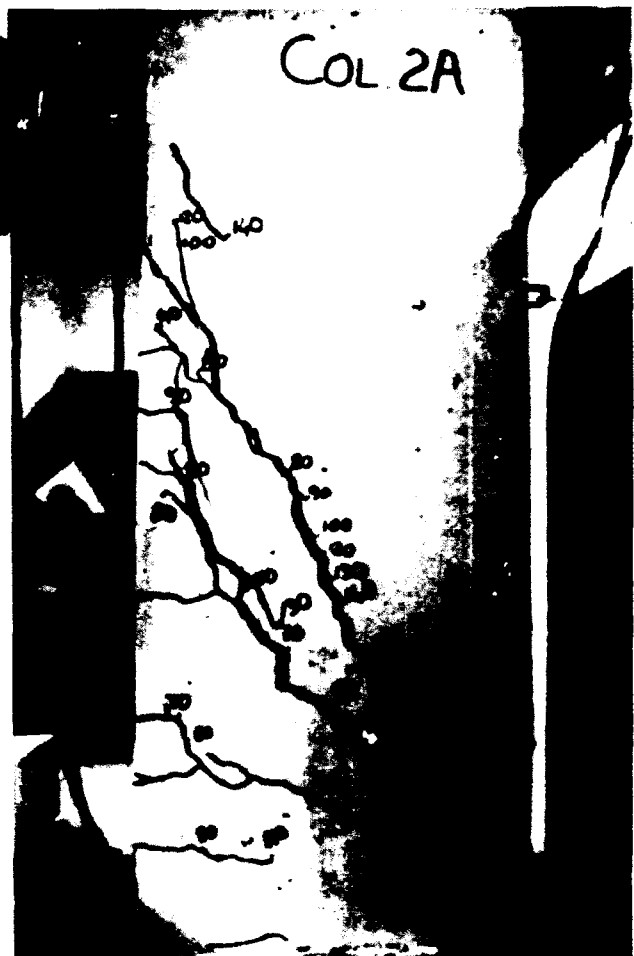
Figure B.43: Crack pattern of Column 2A seen from the other side of the column.
