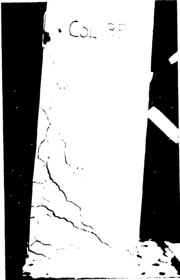
Figure B.74: Crack pattern of Column 3E seen from one side after the static test.
