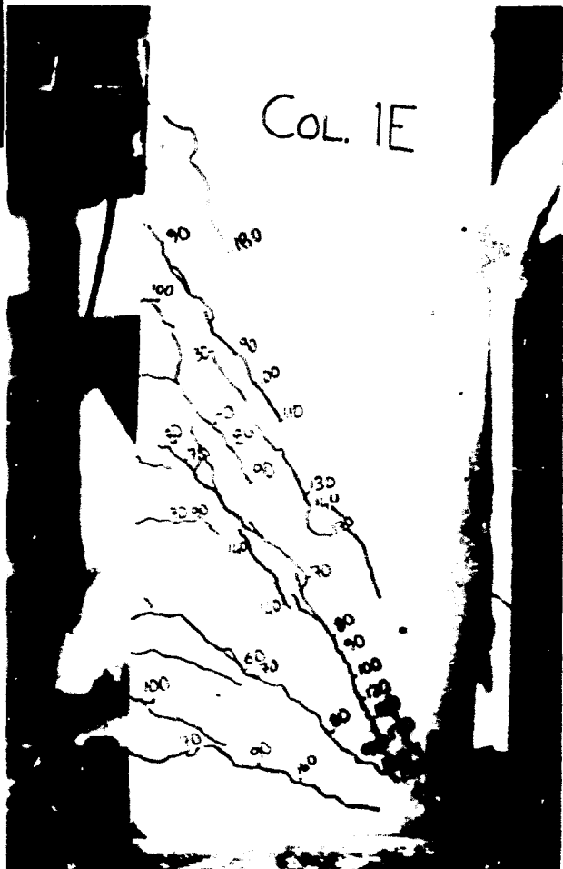
Figure B.35: Crack pattern of Column 1E seen from the other side of the column.
