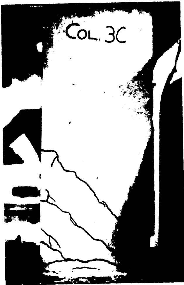
Figure B.64: Crack pattern of Column 3C seen from one side after the impact phase.
