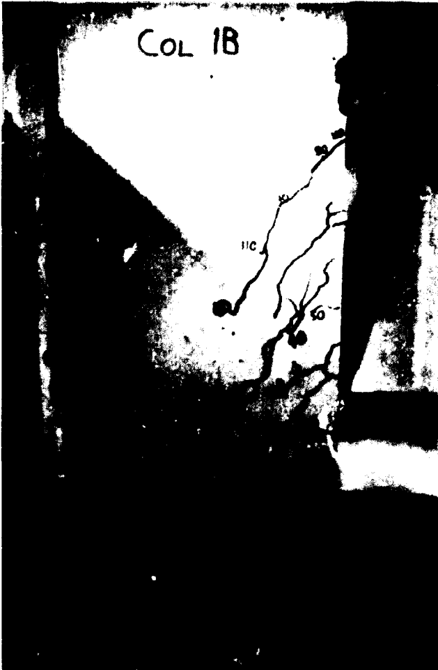
Figure B.28: Crack pattern of Column 1B seen from one side after the static test.
