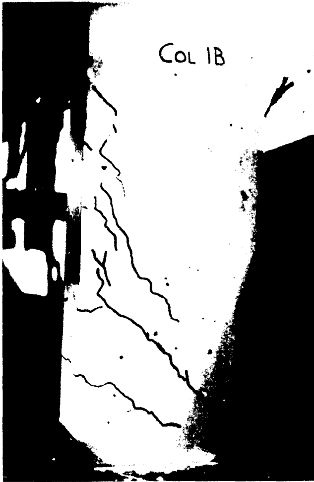
Figure B.26: Crack pattern of Column 1B seen from one side after the impact phase.
