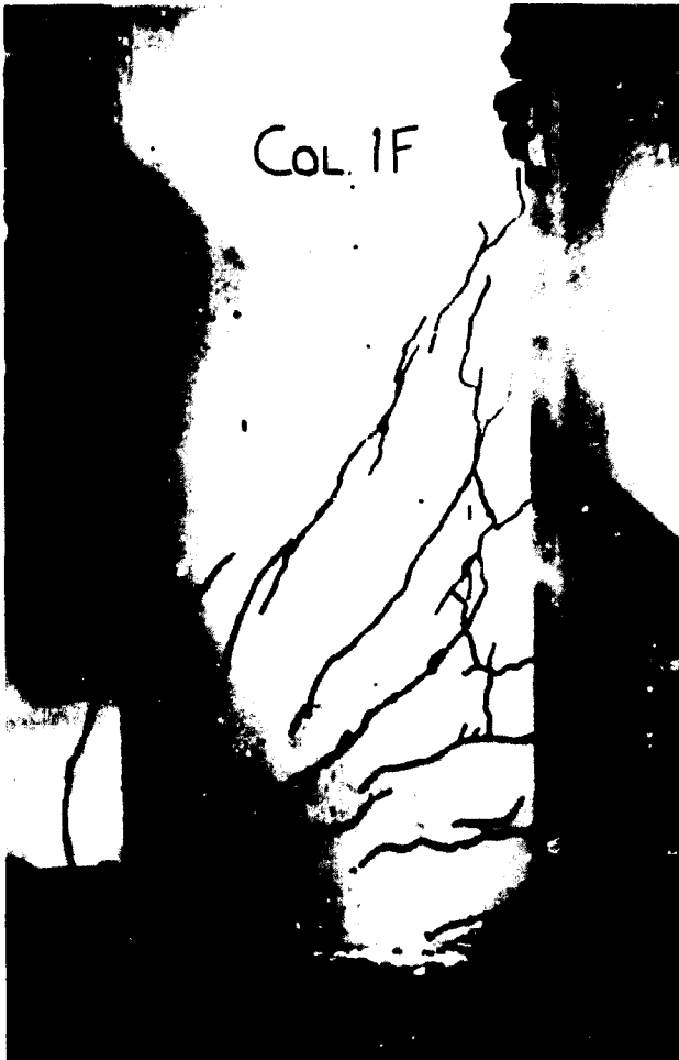
Figure B.36: Crack pattern of Column 1F seen from one side after the impact phase.
