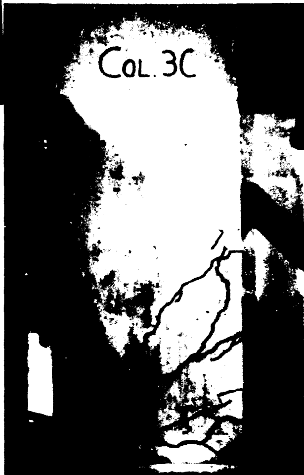
Figure B.65: Crack pattern of Column 3C seen from the other side of the column.
