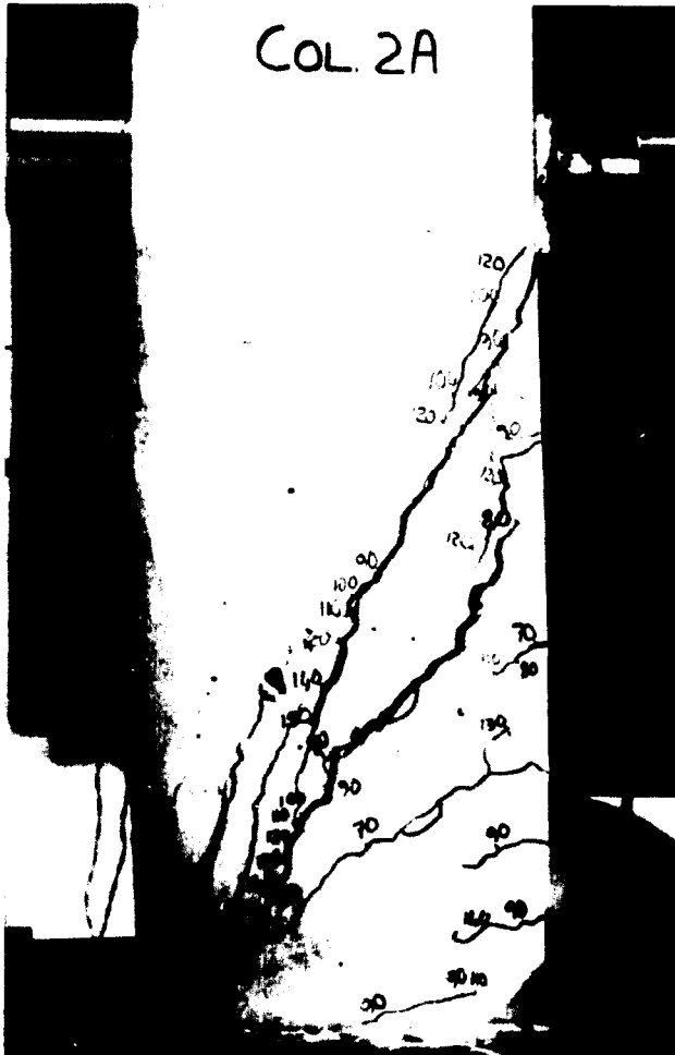
Figure B.42: Crack pattern of Column 2A seen from one side after the static test.
