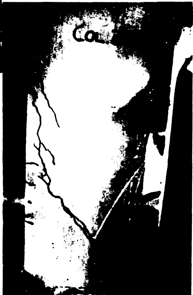
Figure B.45: Crack pattern of Column 2B seen from the other side of the column.
