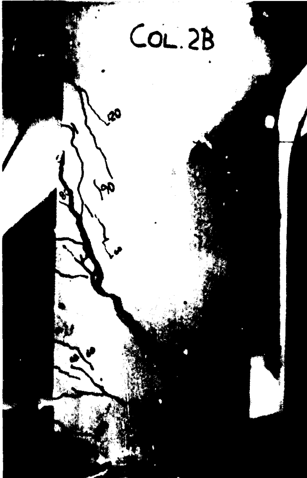
Figure B.46: Crack pattern of Column 2B seen from one side after the static test.
