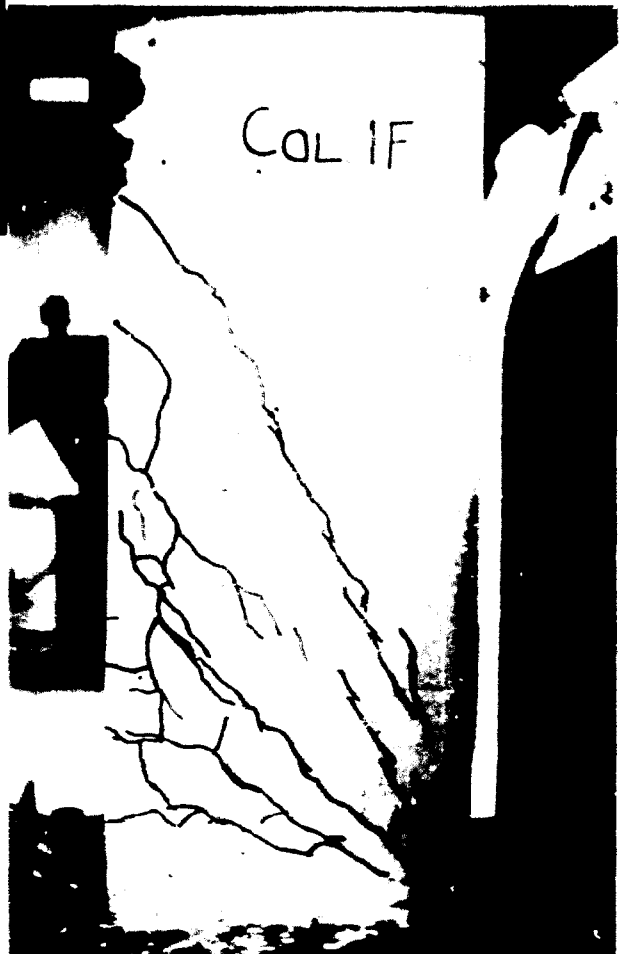
Figure B.37: Crack pattern of Column 1F seen from the other side of the column.
