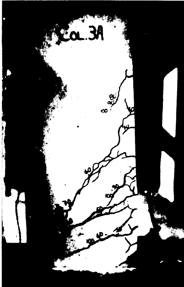
Figure B.58: Crack pattern of Column 3A seen from one side after the static test.
