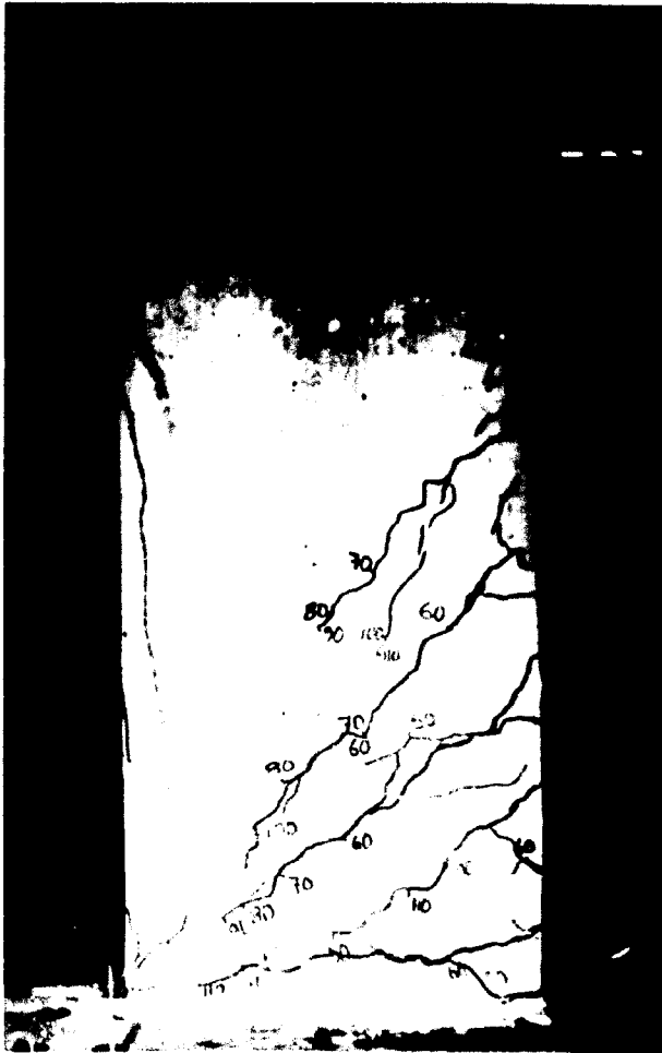
Figure B.88: Crack pattern of Column 5A seen from one side after the static test.
