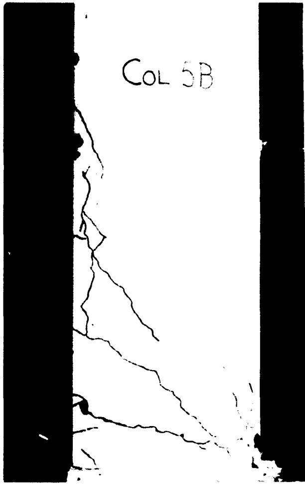
Figure B.90: Crack pattern of Column 5B seen from one side after the impact phase.
