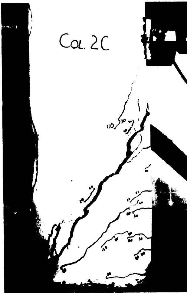
Figure B.50: Crack pattern of Column 2C seen from one side after the static test.
