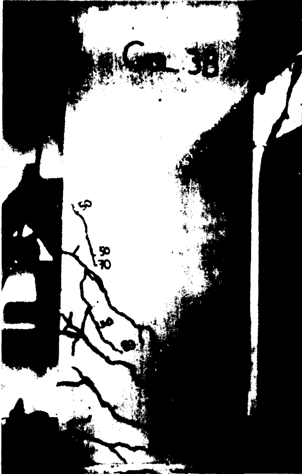
Figure B.62: Crack pattern of Column 3B seen from one side after the static test.
