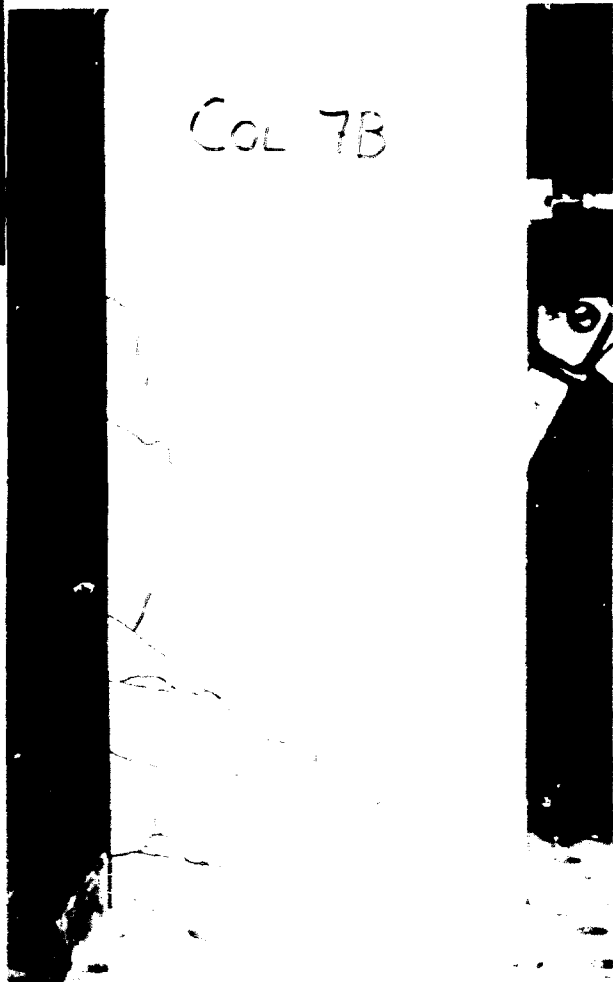
Figure B.111. Crack pattern of Column 7B seen from the other side of the column.
