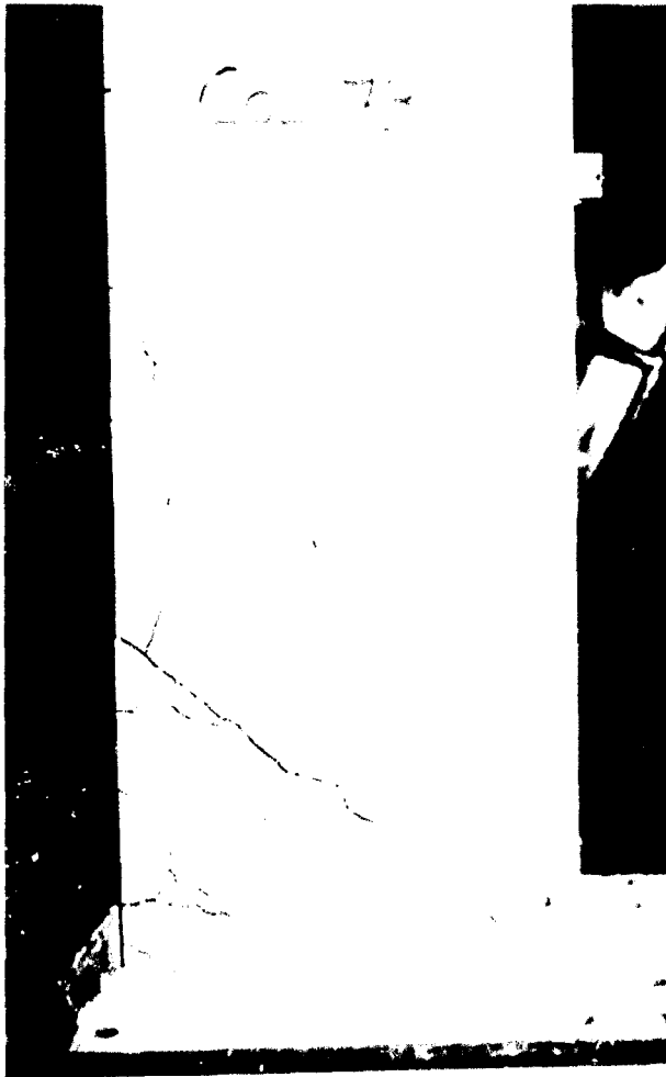
Figure B.112: Crack pattern of Column 7B seen from one side after the static test.
