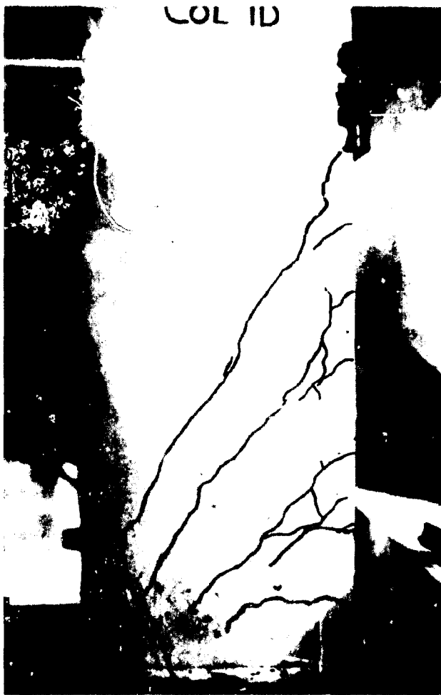
Figure B.52: Crack pattern of Column 1D seen from one side after the impact test.
