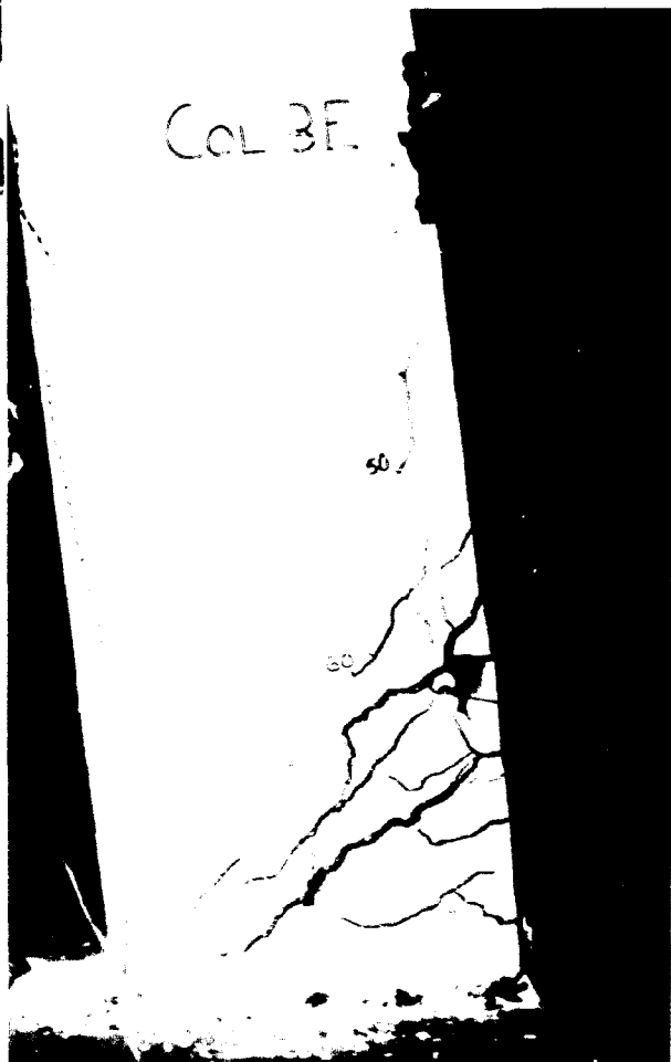
Figure B.75: Crack pattern of Column 3E seen from the other side of the column.
