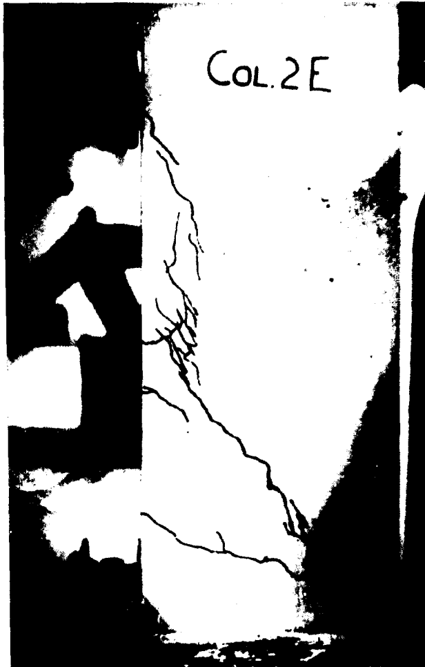
Figure B.54: Crack pattern of Column 2E seen from one side after the impact phase.
