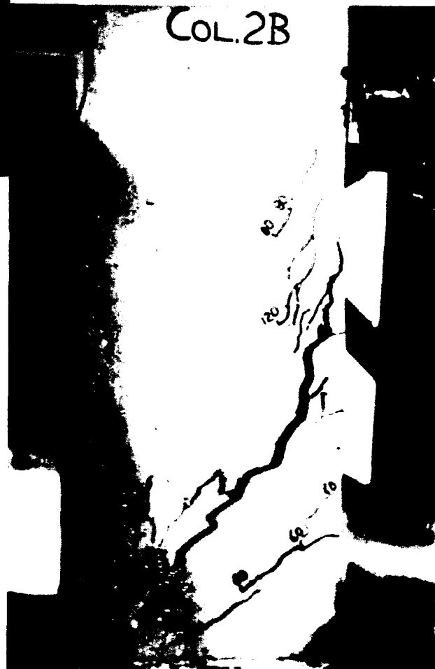
Figure B.47: Crack pattern of Column 2B seen from the other side of the column.
