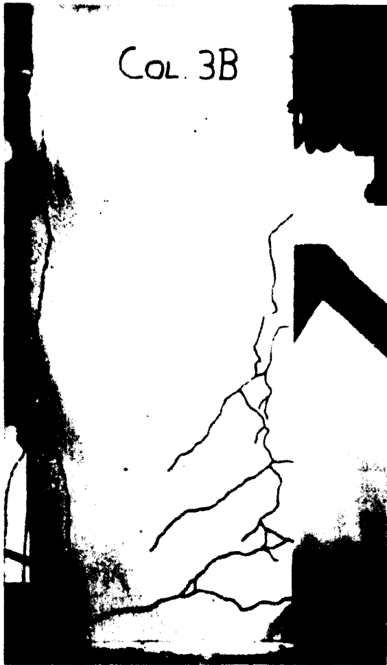
Figure B.60: Crack pattern of Column 3B seen from one side after the impact phase.
