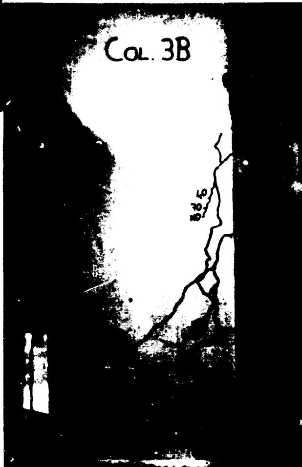
Figure B.63: Crack pattern of Column 3B seen from the other side of the column.
