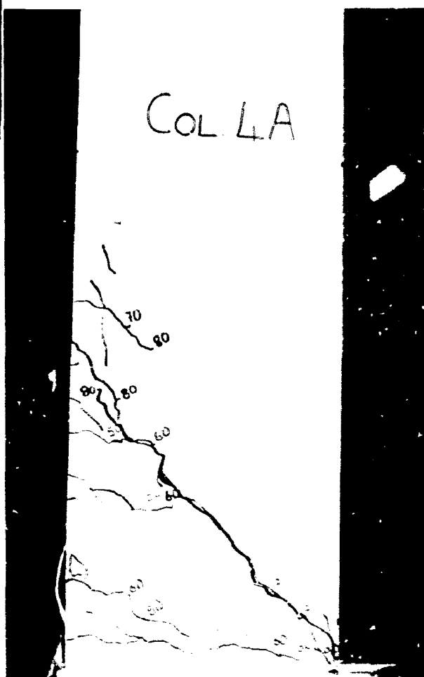
Figure B.77: Crack pattern of Column 4A seen from the other side of the column.
