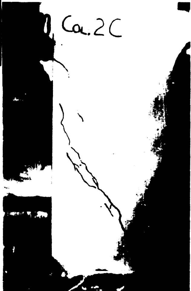
Figure B.49: Crack pattern of Column 2C seen from the other side of the column.
