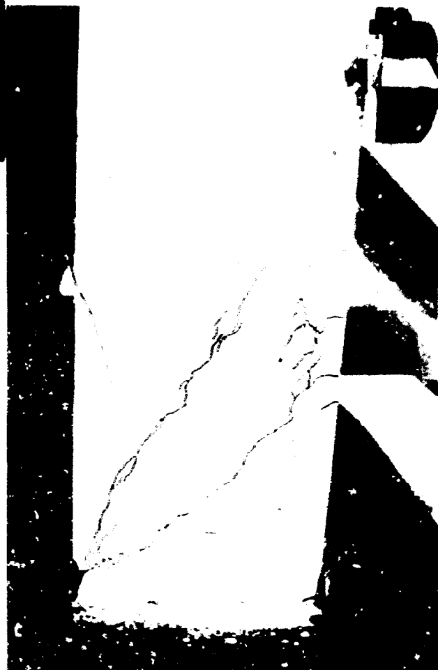
Figure B.31: Crack pattern of Column 1C seen from the other side of the column.
