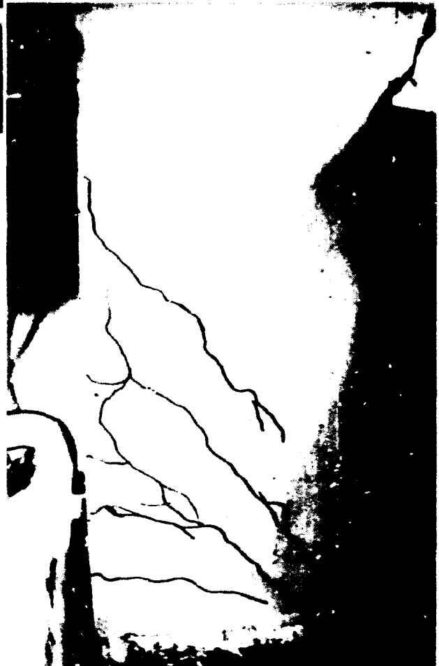
Figure B.53: Crack pattern of Column 1D seen from the other side of the column.
