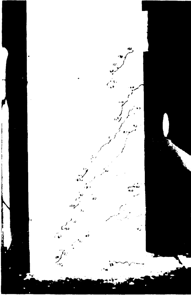
Figure B.24: Crack pattern of Column 1A seen from one side. The numbers next to the lines indicate the horizontal load in kN.
