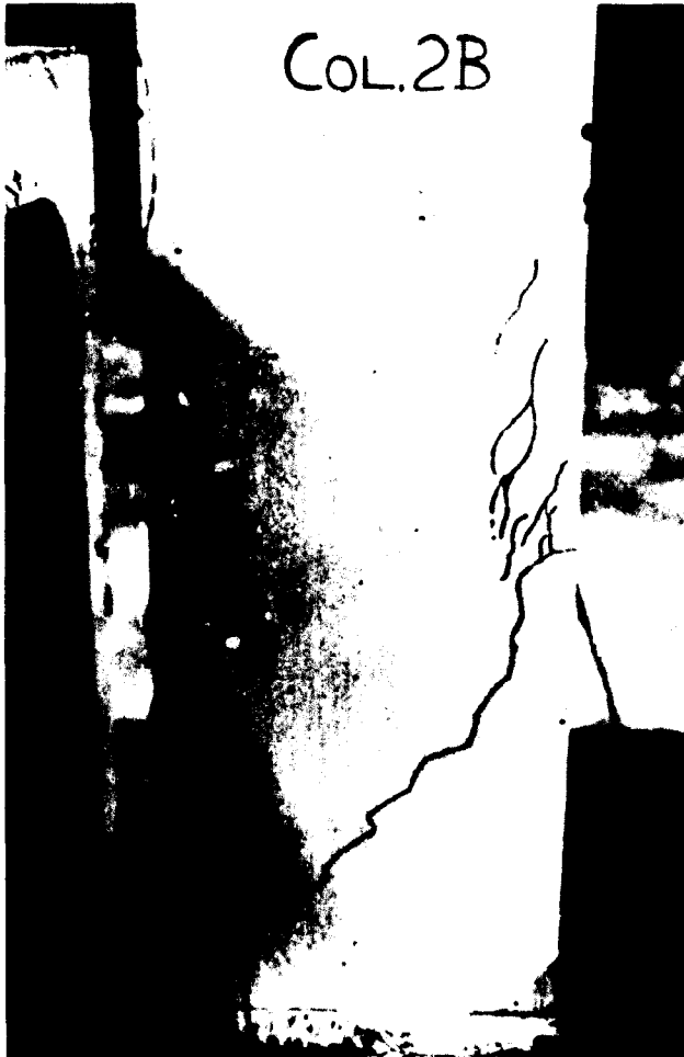
Figure B.44: Crack pattern of Column 2B seen from one side after the impact phase.
