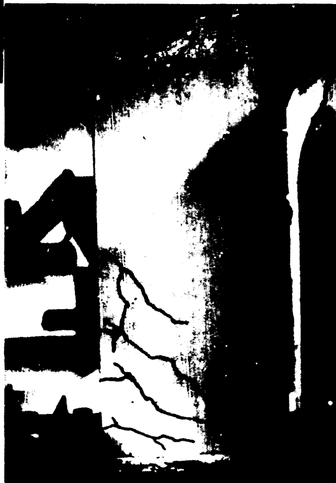
Figure B.61: Crack pattern of Column 3B seen from the other side of the column.
