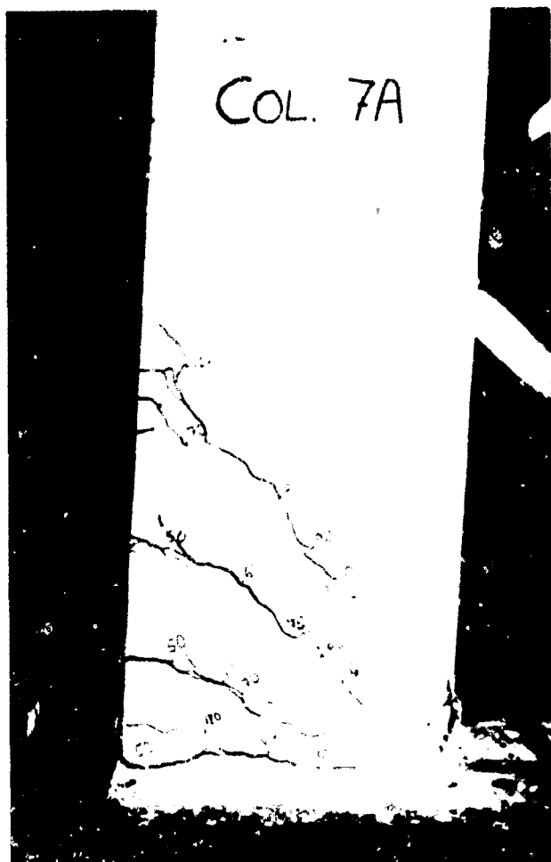
Figure B.108: Crack pattern of Column 7A seen from one side after the static test.
