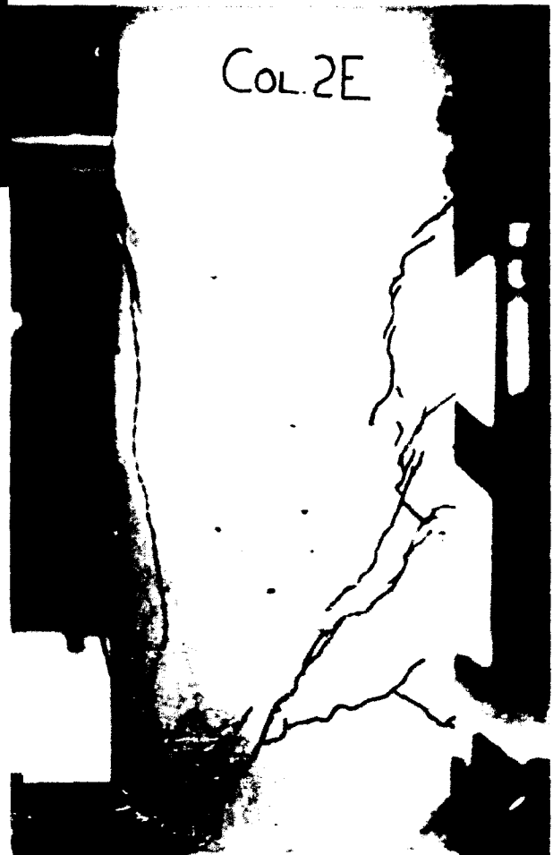
Figure B.55: Crack pattern of Column 2E seen from the other side of the column.
