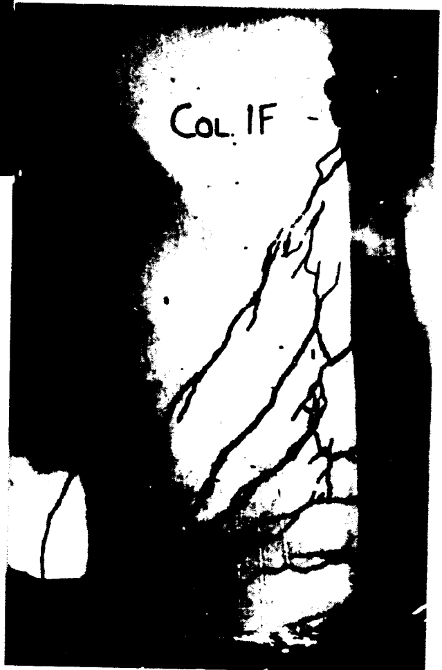
Figure B.39: Crack pattern of Column 1F seen from the other side of the column.
