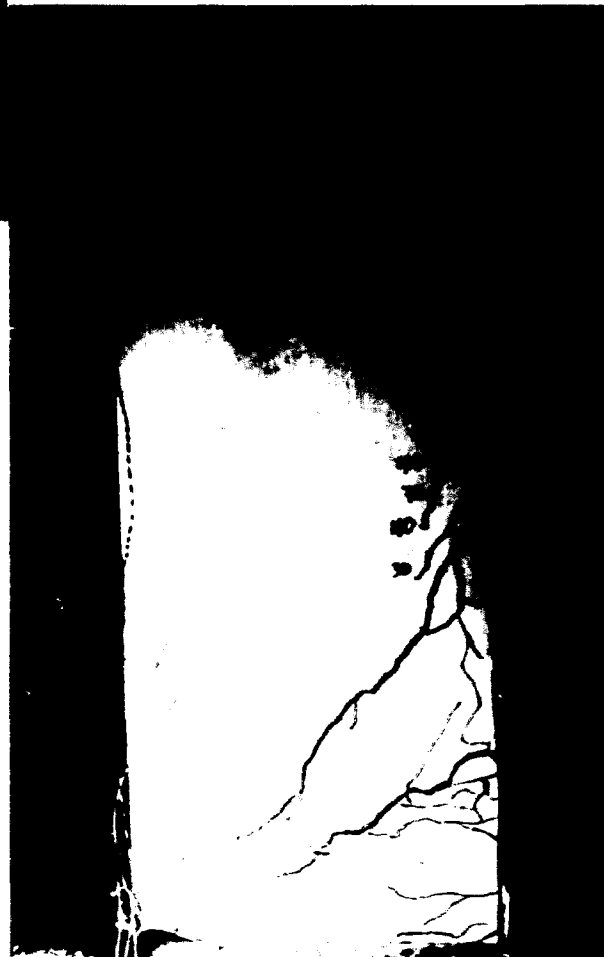
Figure B.85c: Crack pattern of Column 40 seen from the other side of the column.
