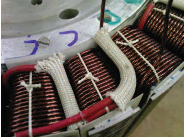
(a) Finished connection
