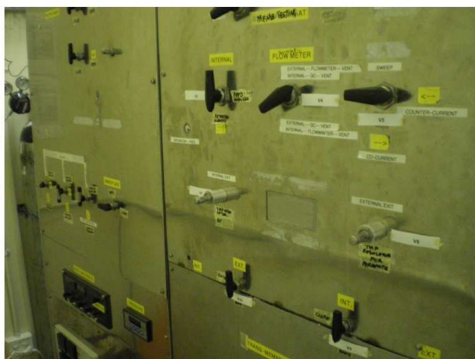
Figure D5: The photograph of the CMR rig at the Department of Process Engineering, Stellenbosch University, South Africa; showing the front view of the control panel.
