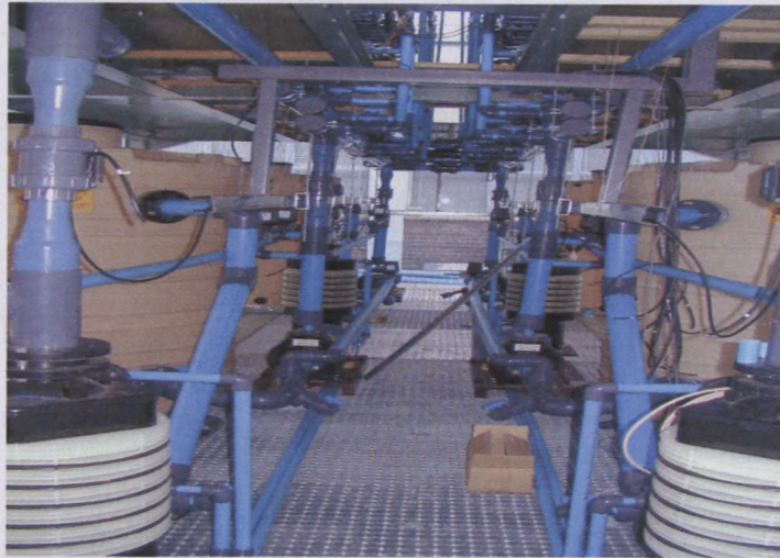
Figure 5.3 Hydraulic sub-system of the VRB
