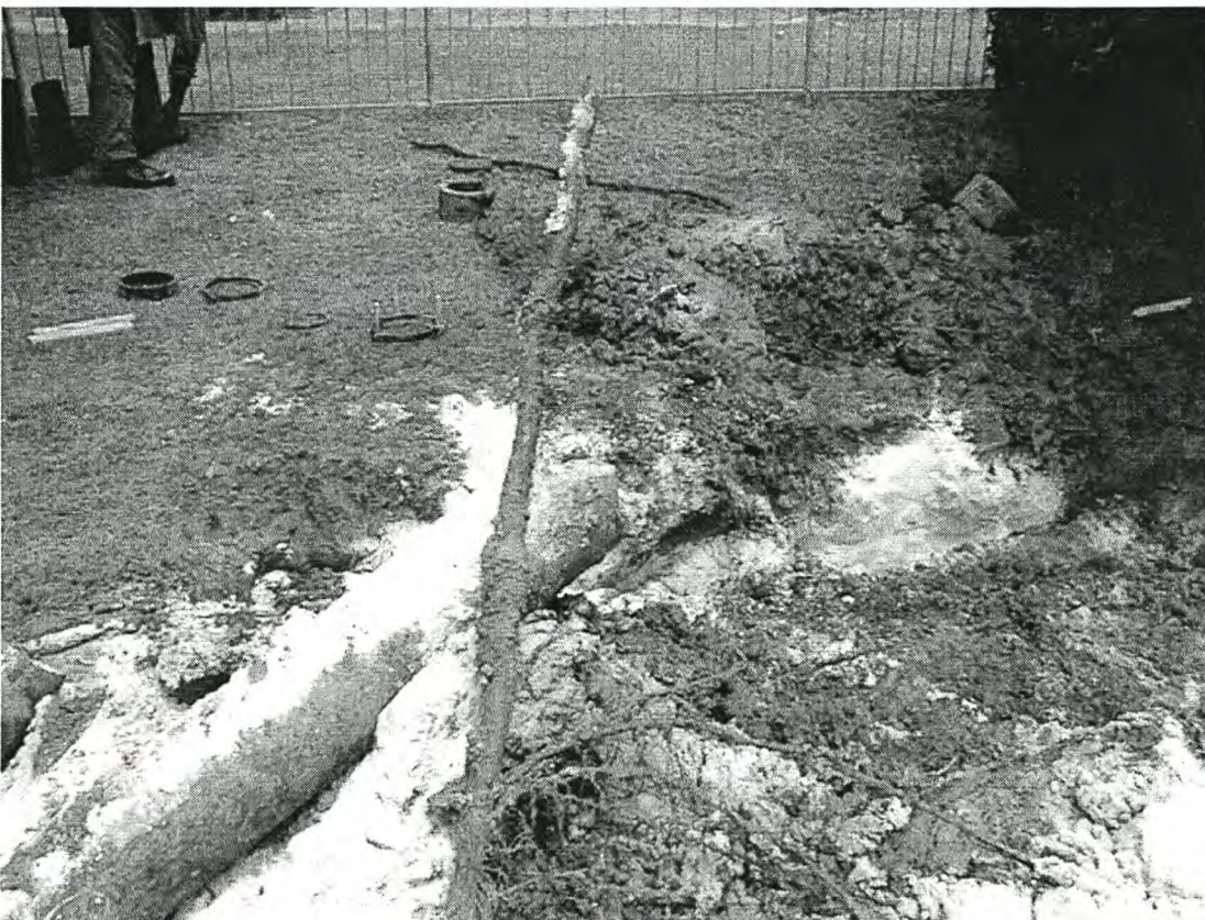
FIGURE 4.2b Pipe break caused by tree roots: Close-up
