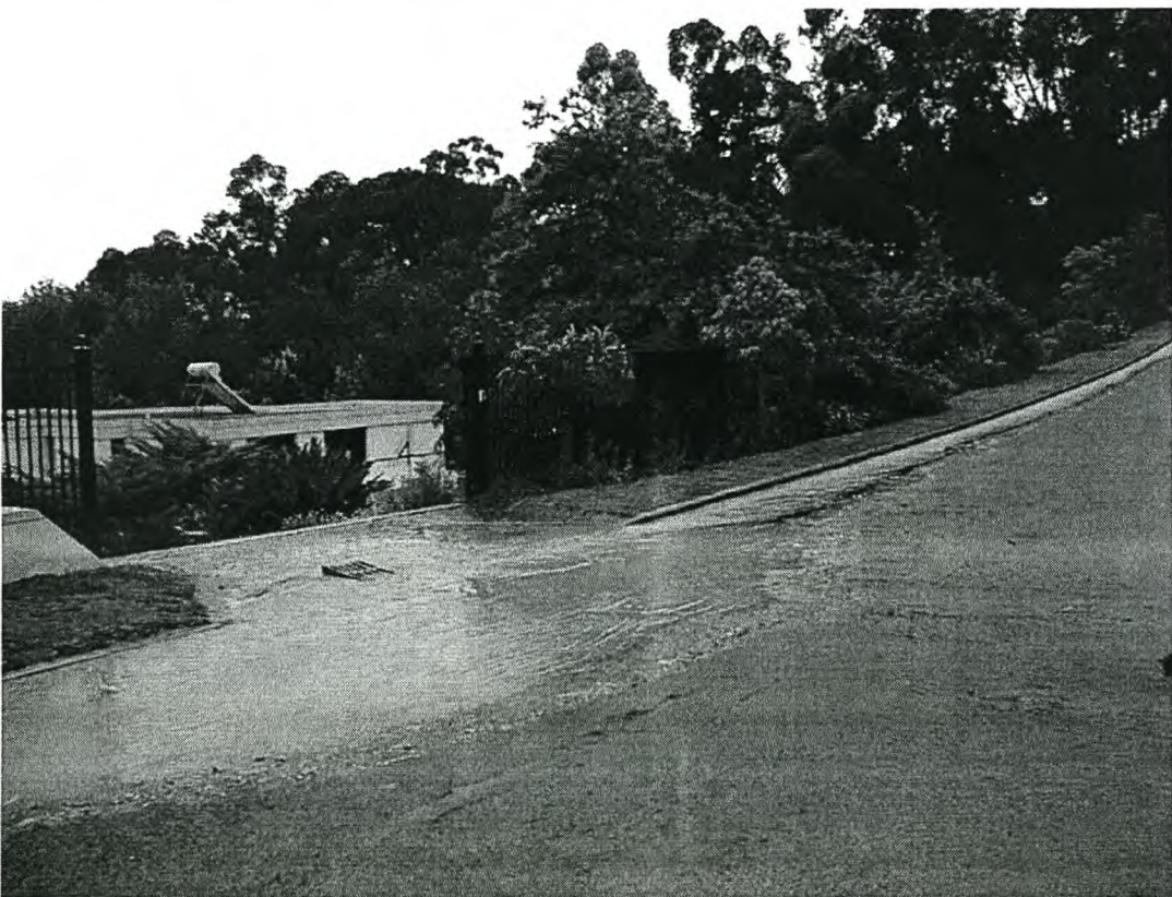
FIGURE 6.22 Stand with very steep cross-slope and pipe break at sidewalk across the street
