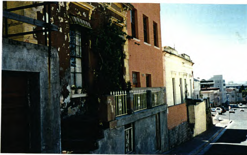
Photo 1. Physical decline in a Cape Town suburb.
