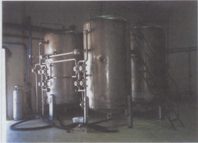
Figure 4.2b Small/4Column Ion Exchange Plant
