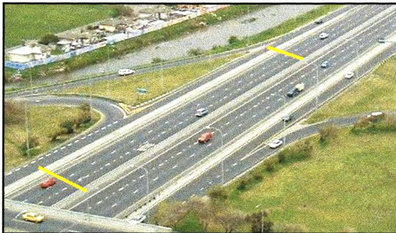
Figure 3.11: Footage for Section 3 (N2 Athlone Power Station)
