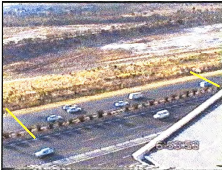
Figure 3.2: Footage for Section 1 (N1 near Century City)
