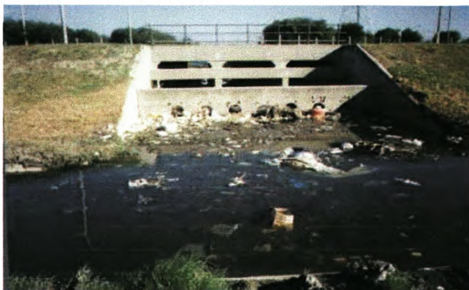
Photo 4.4: Entrance Weir to detention pond
