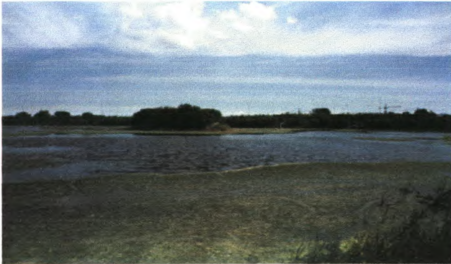
Photo 4.3: Vygekraal Road Detention Pond
