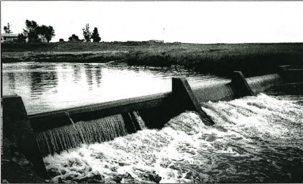
Figure 1.2: Columns between the notches for aeration purposes
