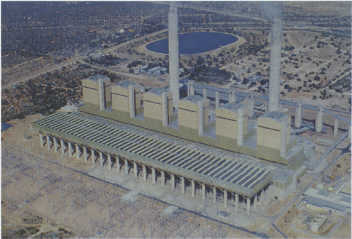
Figure 1.1: Photo of an air-cooled steam condenser system.
