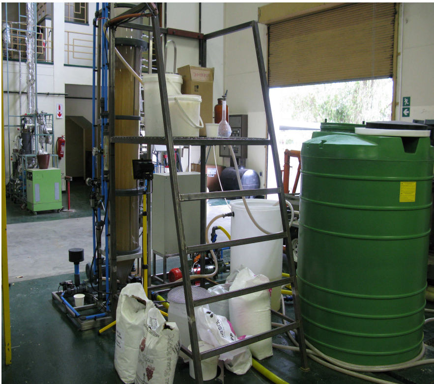
Figure 3.11: Feed water tank and platform ladder.
