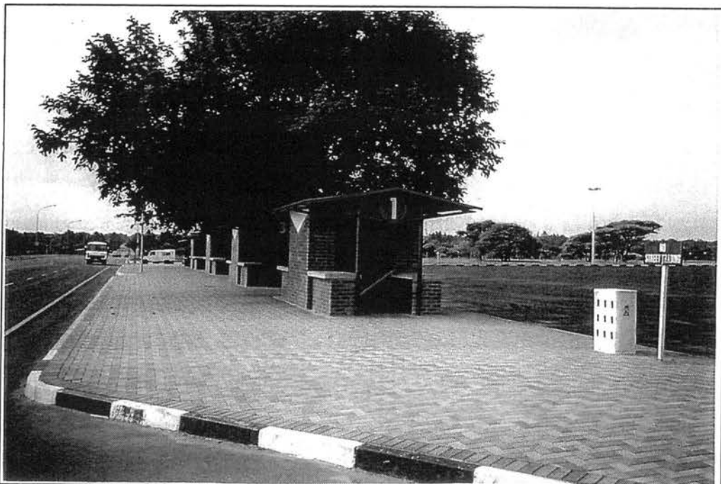
PLATE 7.2: LOCK-UP STREET TRADING FACILITIES AT THE PIETERSBURG SPORTS STADIUM
