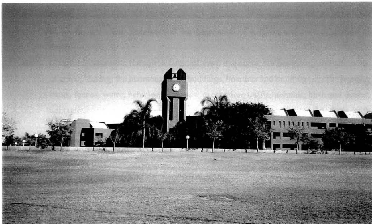
PLATE 3.4: GOVERNMENT COMPLEX OF FORMER LEBOWA IN LEBOWAKGOMO, 1998
