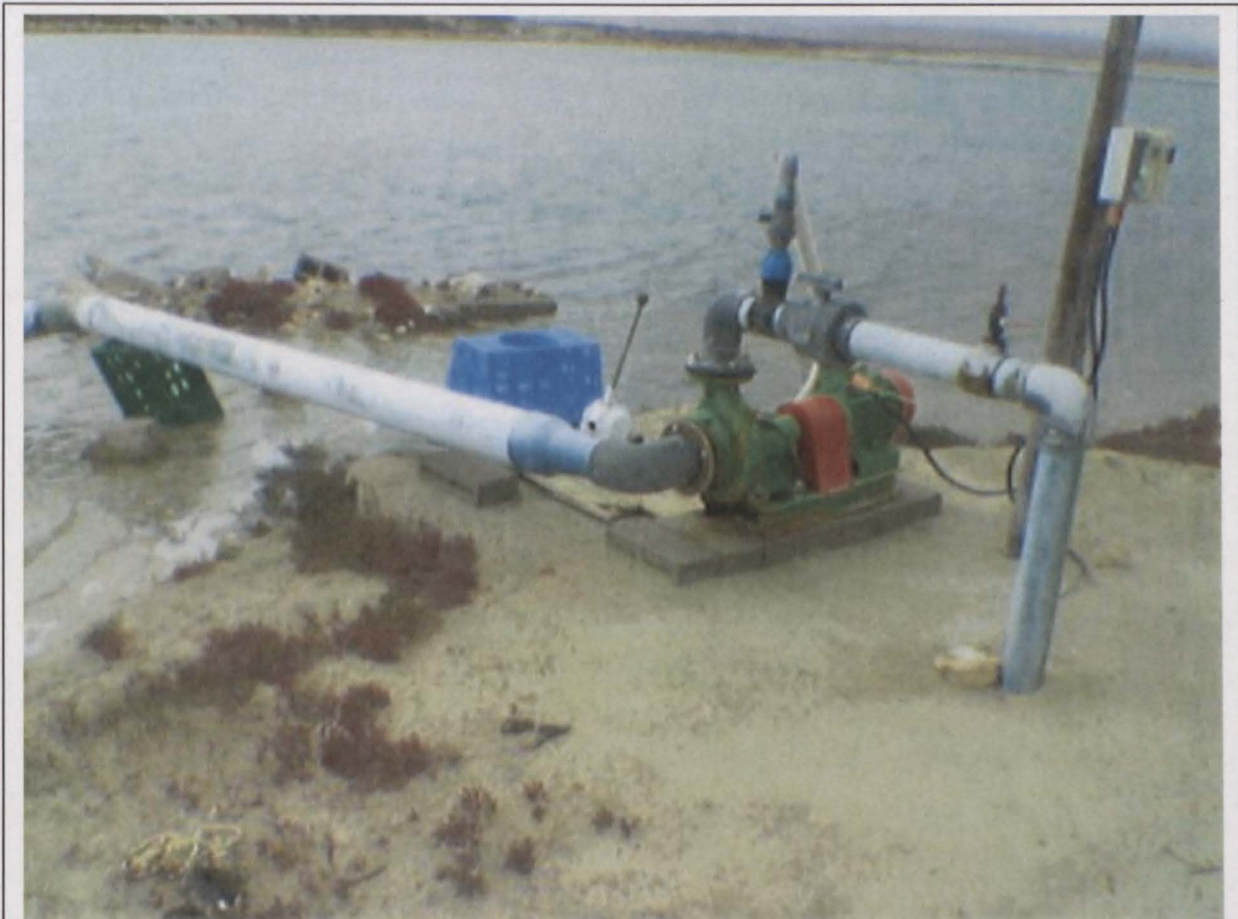
Figure 14 Pump the supply of water from the cultivation ponds to the nursery.
