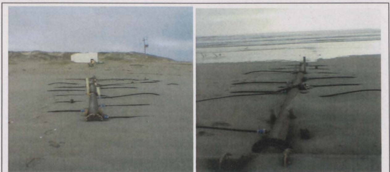
Figure 11 The inlet manifold at the low water level with the pump house in the background.
