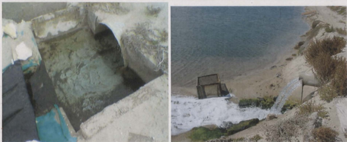
Figure 13 Sump showing culvert to pond and a pipe supply to another pond
