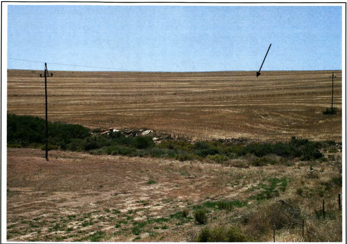
Figure 2.3: Power line against a golden yellow background of the harvested fields. The arrow shows section of the power line that is not visible.
