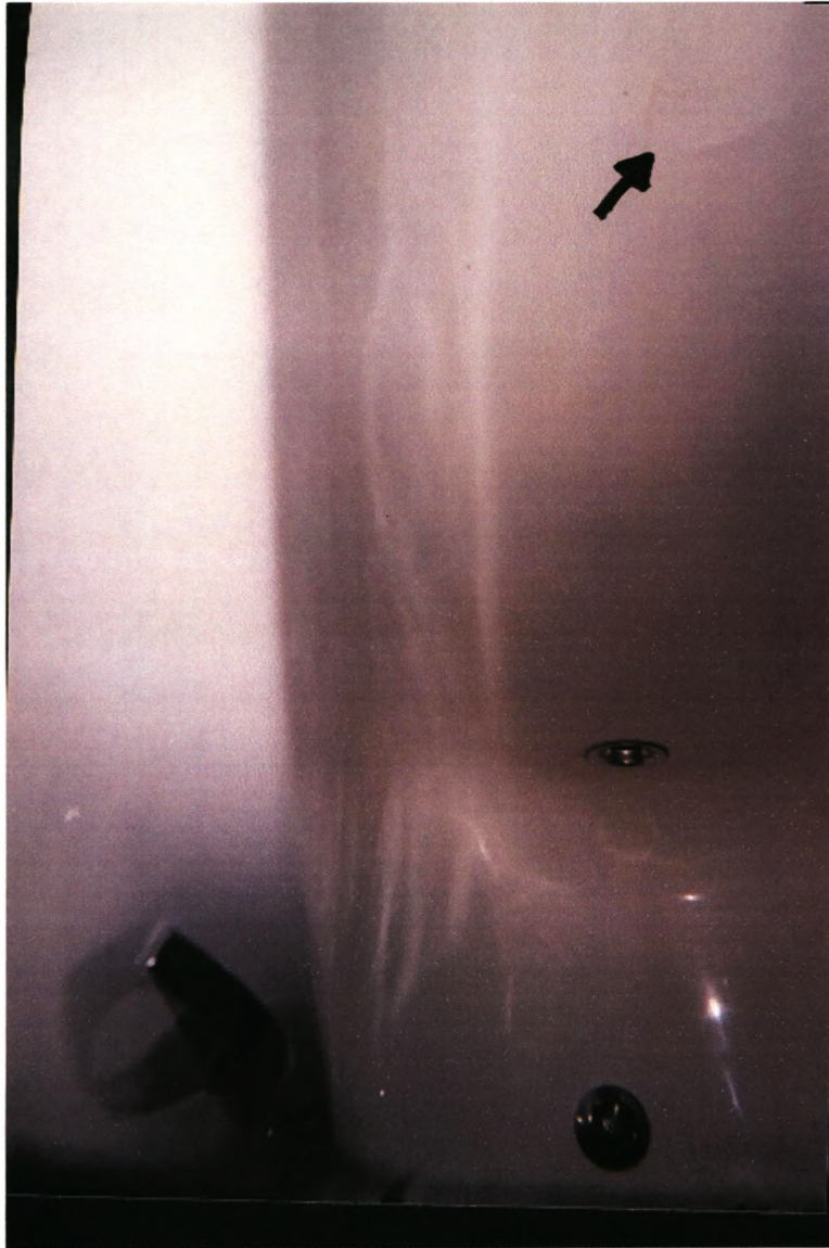
Picture 5.1 indicating cracking bath
