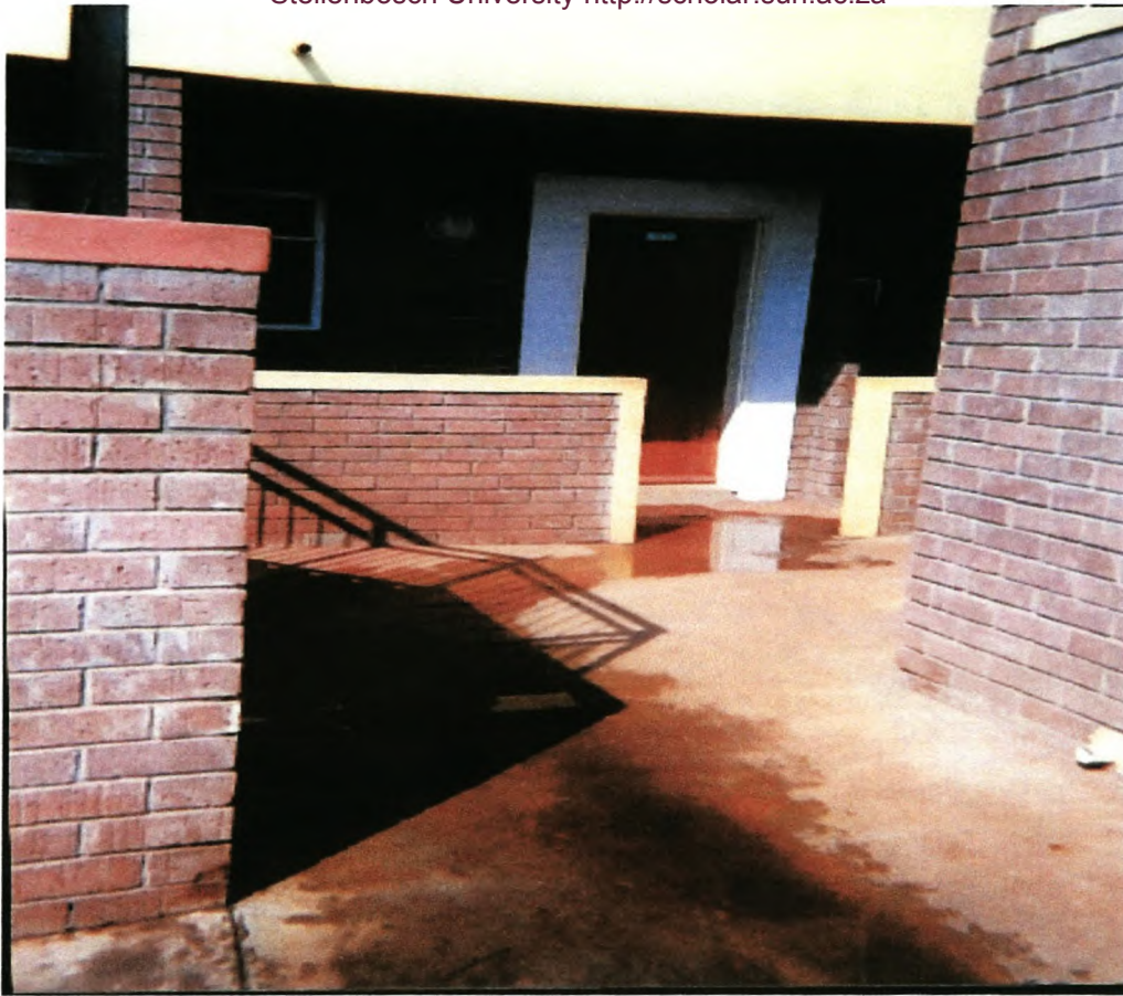
Picture 5.10 indicating the water leakage outside the unit
