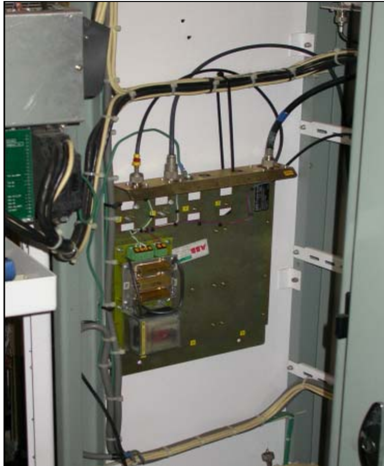
Photograph 4.1 Installation of a measurement hybrid
