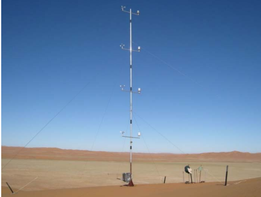
Figure 14: The wind mast
