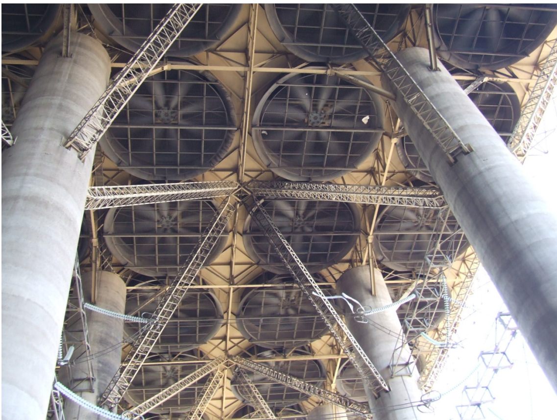
Figure 1.4 View from below ACC fan array showing rows of axial cooling fans
