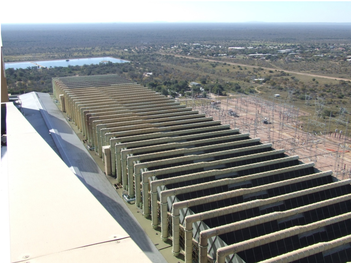
Figure 1.1 Air-cooled condenser (ACC) at the largest dry-cool power station in the world
