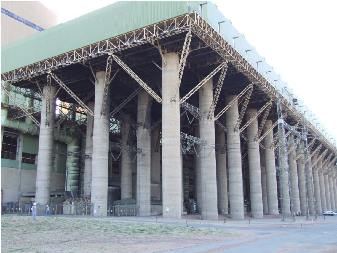
Figure 1.3 Fan array platform of the ACC
