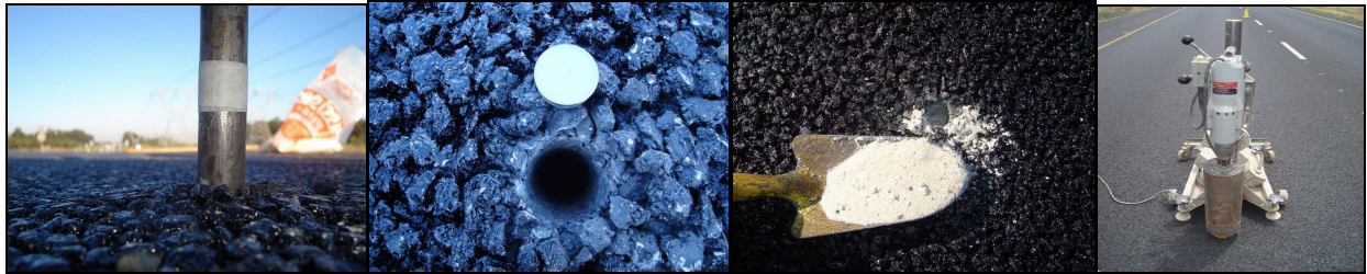
Figure 5.10 Installation of i-buttons on N7 highway for temperature & relative humidity measurements
