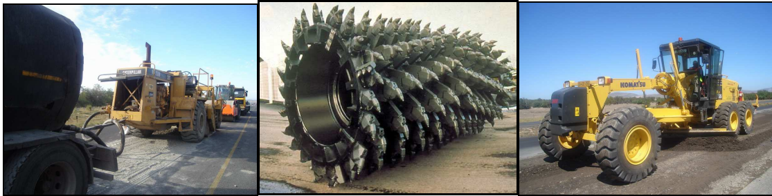
Figure 5.2 Schematic process of N7 CIPR construction project, April 2007
