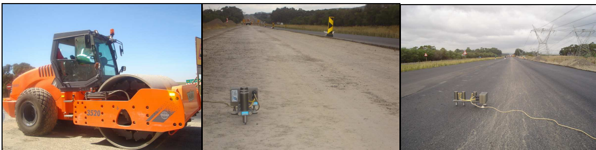
Figure 5.13 Field compaction using high energy steel rollers and the relative impact on resilient modulus
