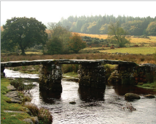
Figure 4: Granite slab used as a foot bridge, Postbridge, Dartmoor, UK.
