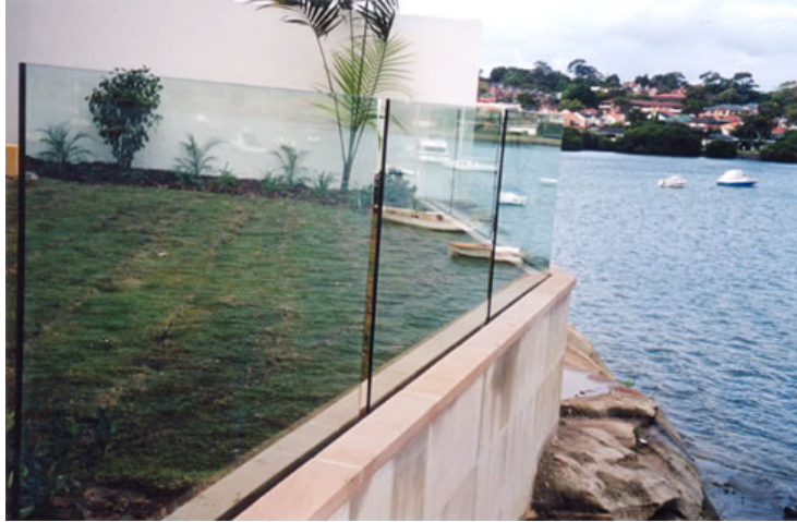
Figure 5.4. Continuously supported freestanding glass balustrade
