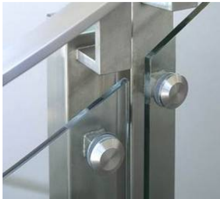
Figure 5.12. Typical glass point support Figure 5.13. Ball and socket joint (Button)
