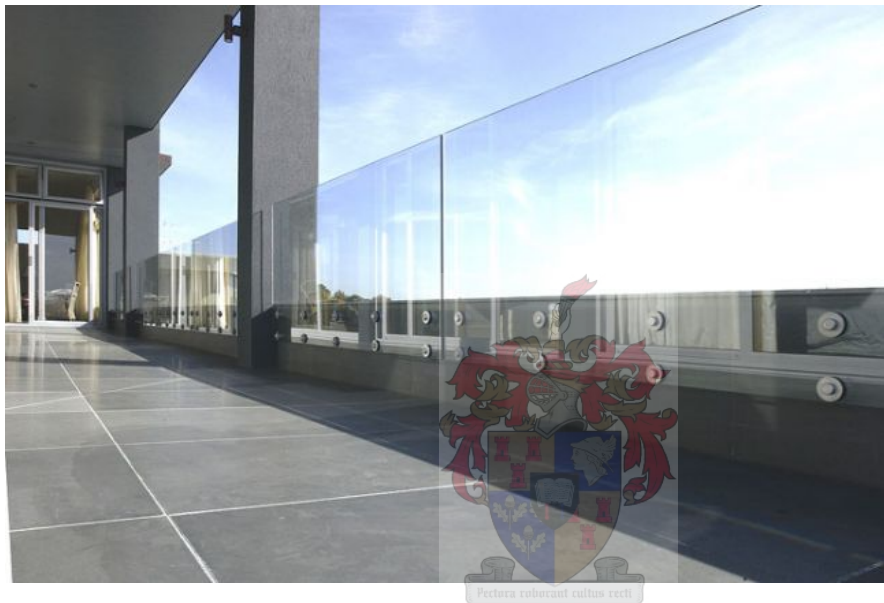
Figure 1.3 Example of freestanding glass balustrade
