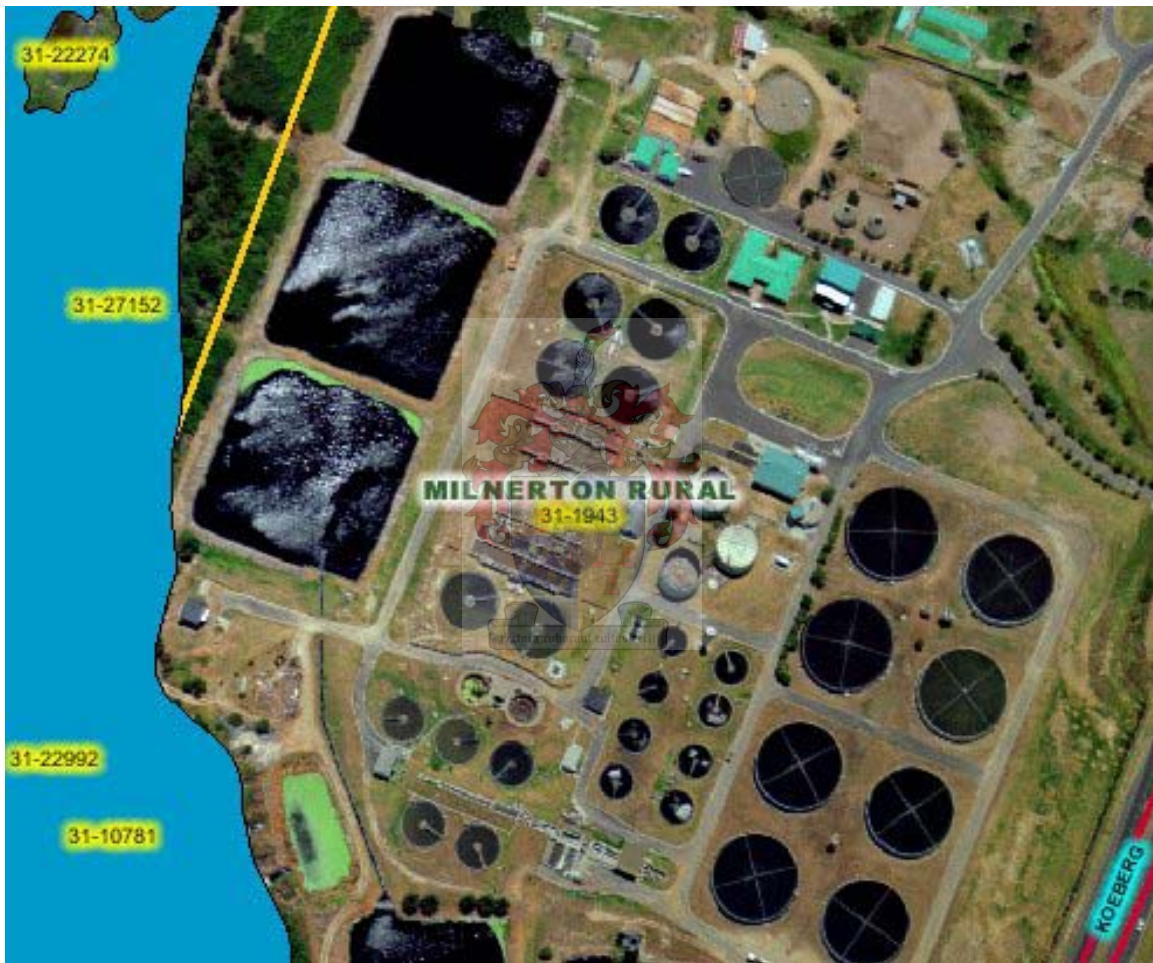
Fig. 2.1 Aerial view of Potsdam WWTW
