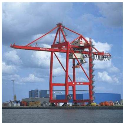
(a) A ship-to-shore container crane. There are various sizes of these cranes, the more popular ones being the Panamax, Post-Panamax and Super Post-Panamax sized cranes [182].
