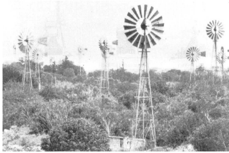
Figure 1.1: Classical windmill used for water pumping.
