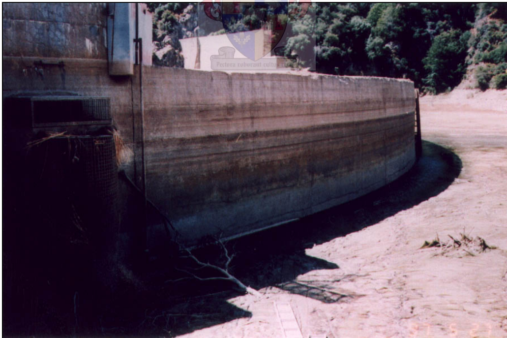
Figure 5-55: Matilija dam wall and sediment deposits, (Matilija Coalition, 2002)
