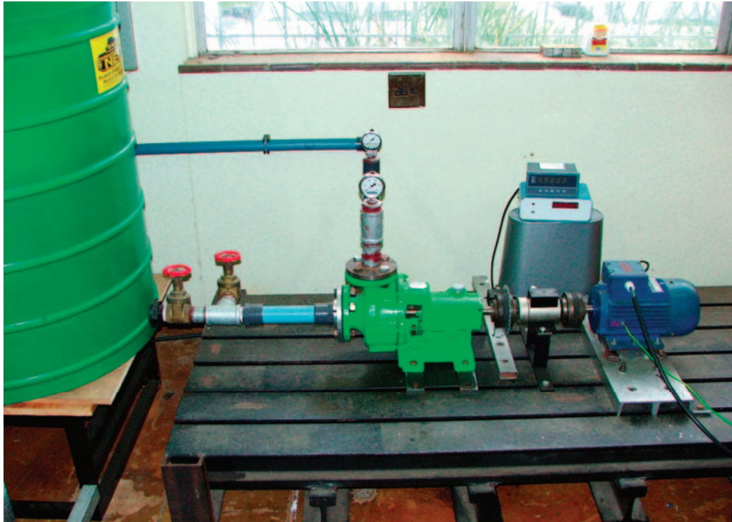
Figure 29: Test setup at the bottom tank of the re-circulating pump system. The torque and speed sensors at the shaft between the 2.2 kW induction motor and centrifugal pump can be observed.
