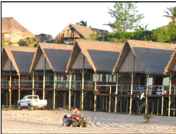
Figure 3.16 An accommodation establishment in Barra showing the use of natural building materials
