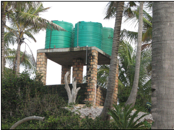
Figure 3.11 Tanks storing borehole water in Guinjata
