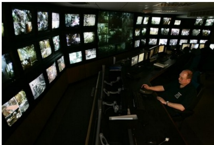
Figure 1.1: Surveillance monitor room
