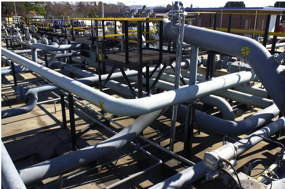
Figure 1.1: An example of a petrochemical plant
