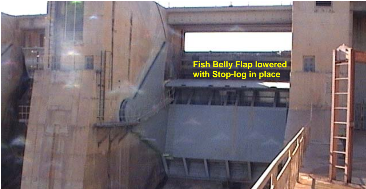
Figure 2.3-4: Elandsdrift Dam Radial Gate with Fish Belly Flaps lowered and Stop-Log in Place
