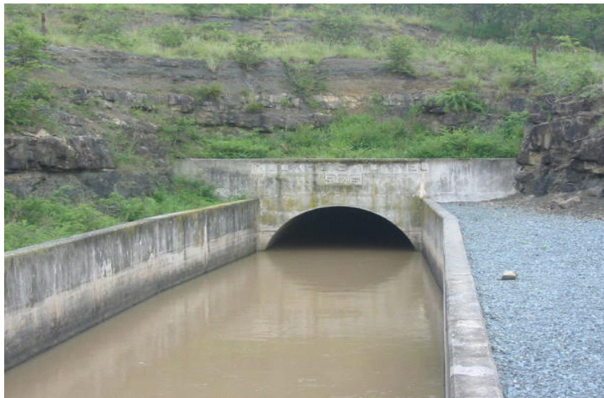
Figure A-13: Cookhouse Tunnel Outlet on the Little Fish Canal
