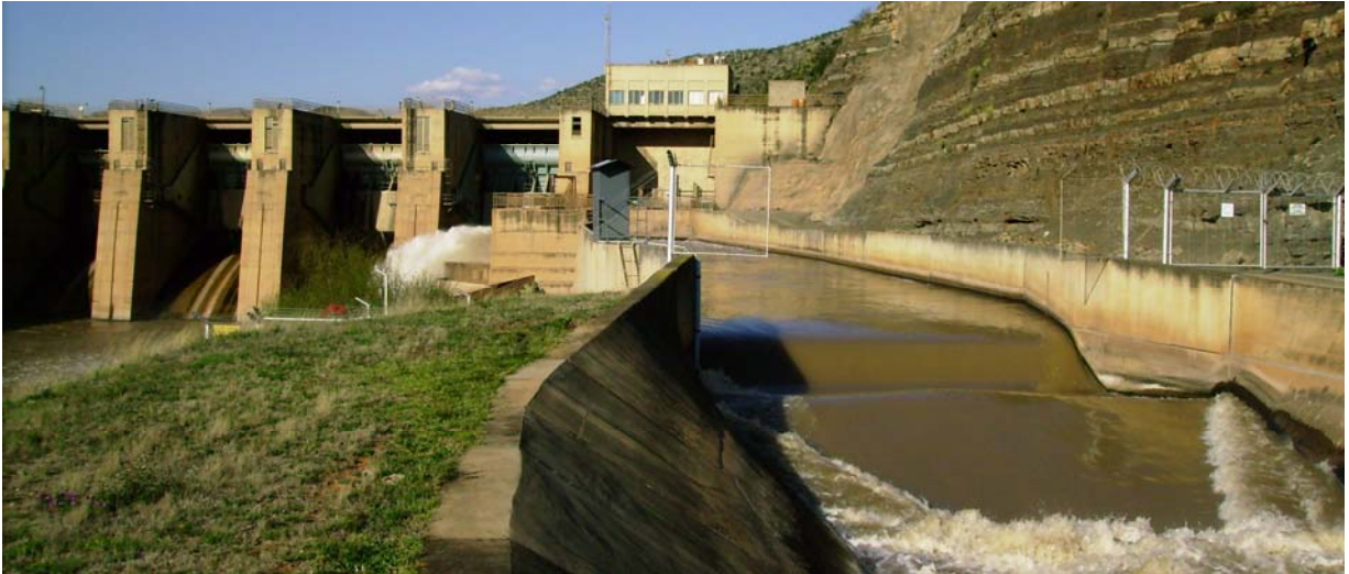
Figure 5.10-11: Elandsdrift Dam Showing the Flow Gauging Station on the Little Fish Canal as well as the Four Radial Flood Gates
