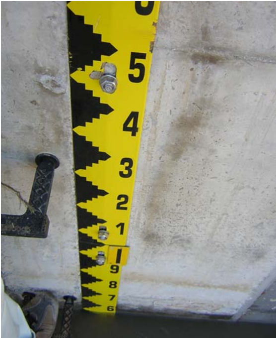
Figure 7.1-3: Gauge Plate on the Weir
