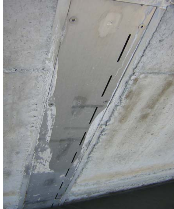
Figure 7.1-4: Slotted Plate over the Chamber
