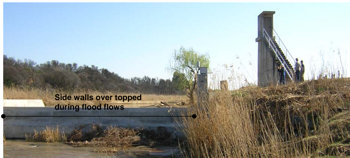
Figure 7.1-2: Downstream View of the Side Walls of Waaikraal Weir
