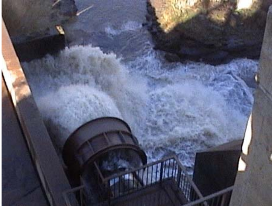
Figure 2.6-2: One of the Sleeve Valves to Release Flow to the Little Fish River at De Mistkraal Dam
