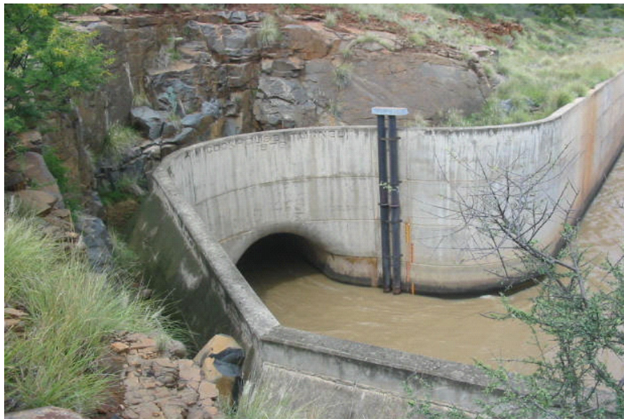
Figure A-11: Cookhouse Tunnel Intake on the Little Fish Canal
