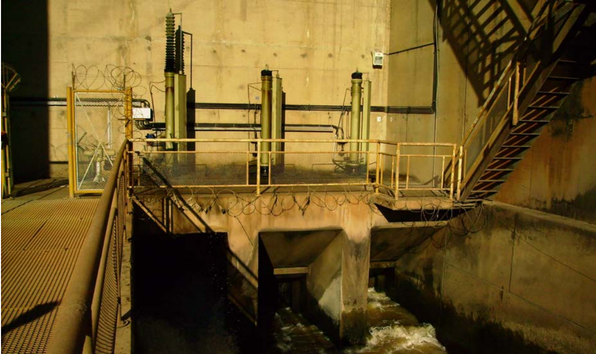
Figure 2.3-3: Elandsdrift Dam Vertical Sluice Gates to Canal
