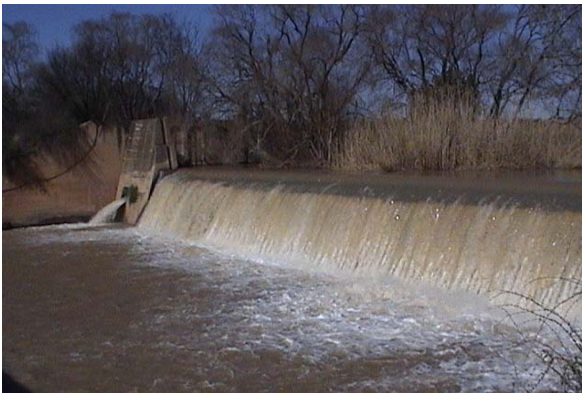
Figure 5.3-2: Flow over the Diversion Weir at Katkop on the Groot Vis River
