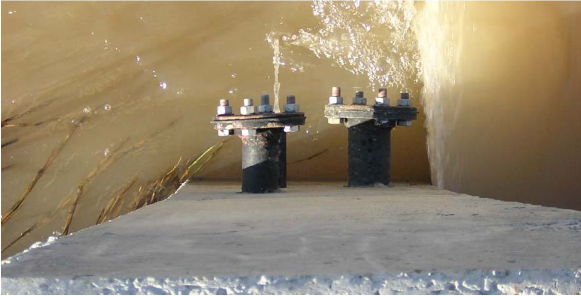
Figure 7.1-5: Water from EC Meter trickling out for the End of the Side Wall
