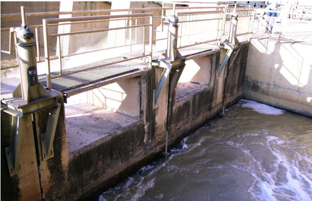
Figure 2.3-7: Elandsdrift Dam Vertical Sluice Gates from Canal to Groot Vis River
