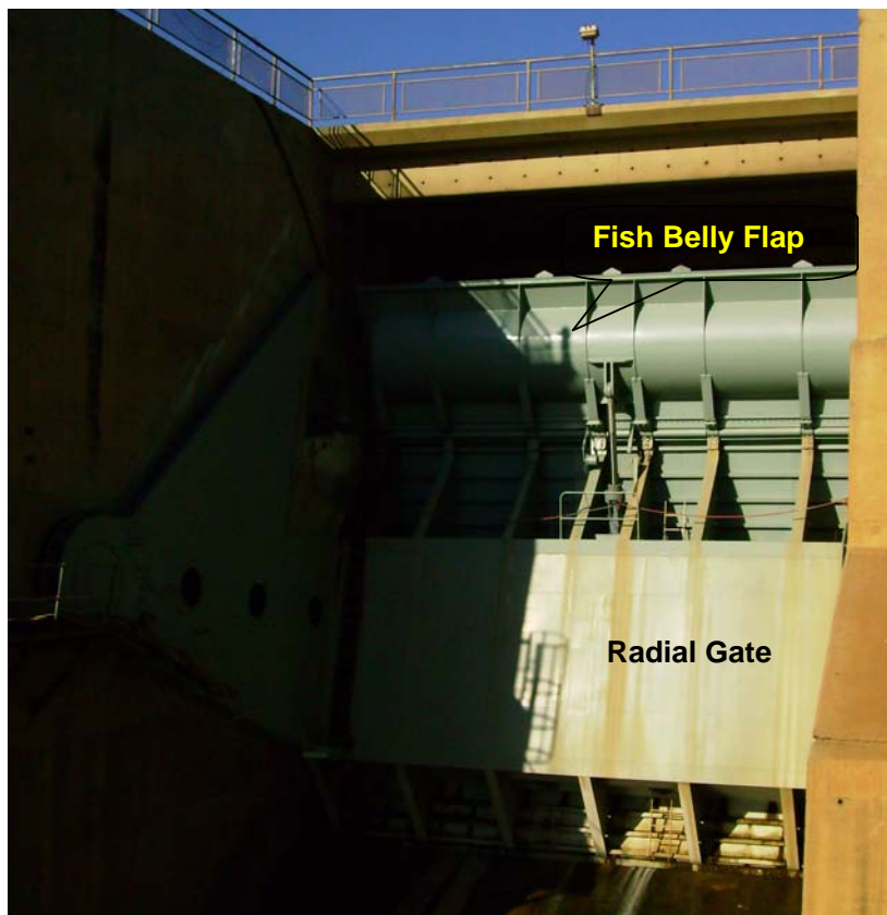
Figure 2.3-5: Close up Picture of the Fish Belly Flap on the Radial Gates of Elandsdrift Dam
