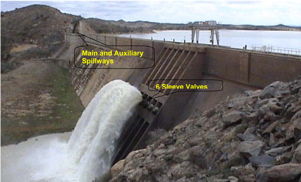
Figure 2.8-2: Darlington Dam Showing the Position of the Diversion Works and Spillways
