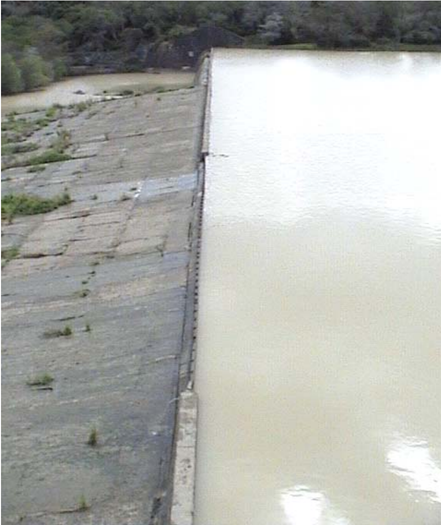
Figure 2.9-1: A View of the Weir at Korhaansdrift on the Sundays River
