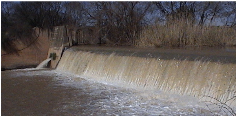
Figure A-6: Katkop Weir on the Groot Vis River
