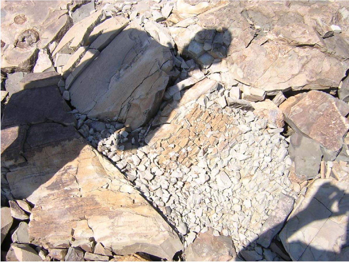
Figure 4.4-1: The Weathering of the Riprap Protection on the Grassridge Dam Embankment
