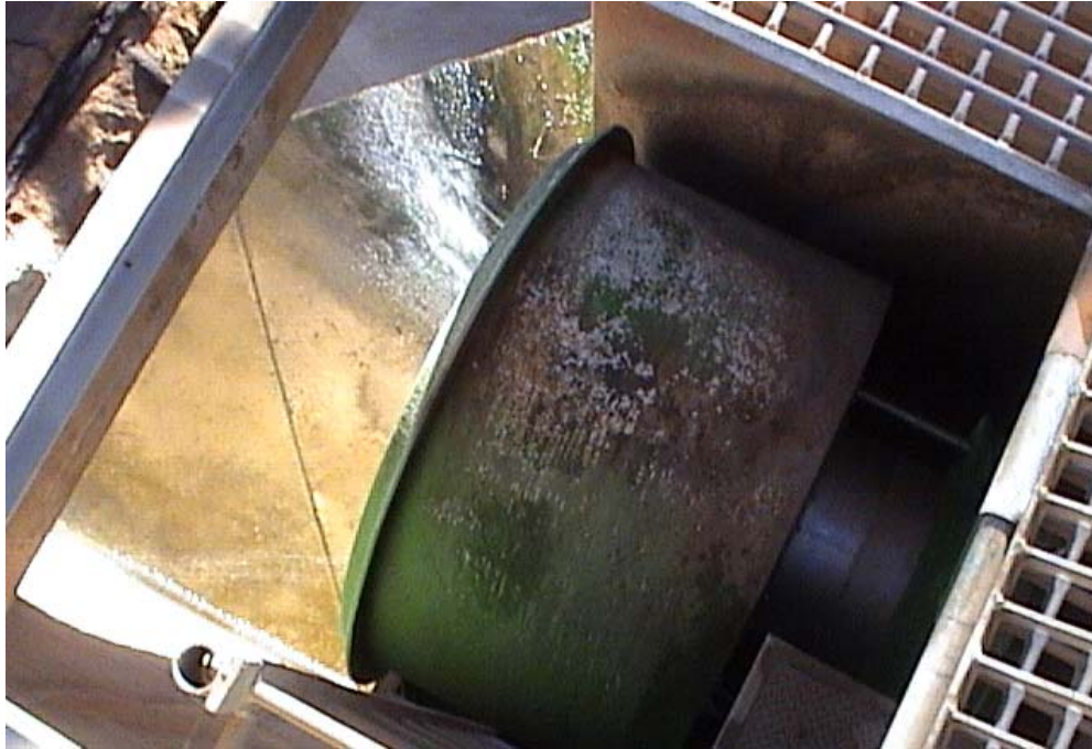
Figure 2.3-6: A Close up Picture of one of three Sleeve Valves to Release Water from Elandsdrift Dam to the Groot Vis River
