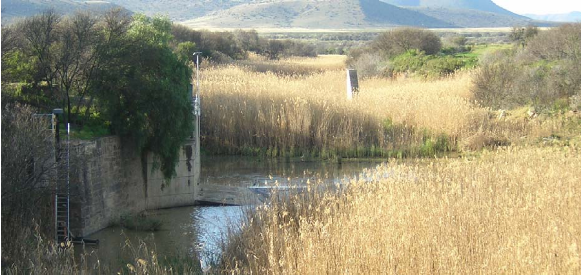
Figure 7.1-7: Tarka Bridge Weir showing the Reeds that have grown on the sediments that have been deposited on the Banks and Behind the Weir
