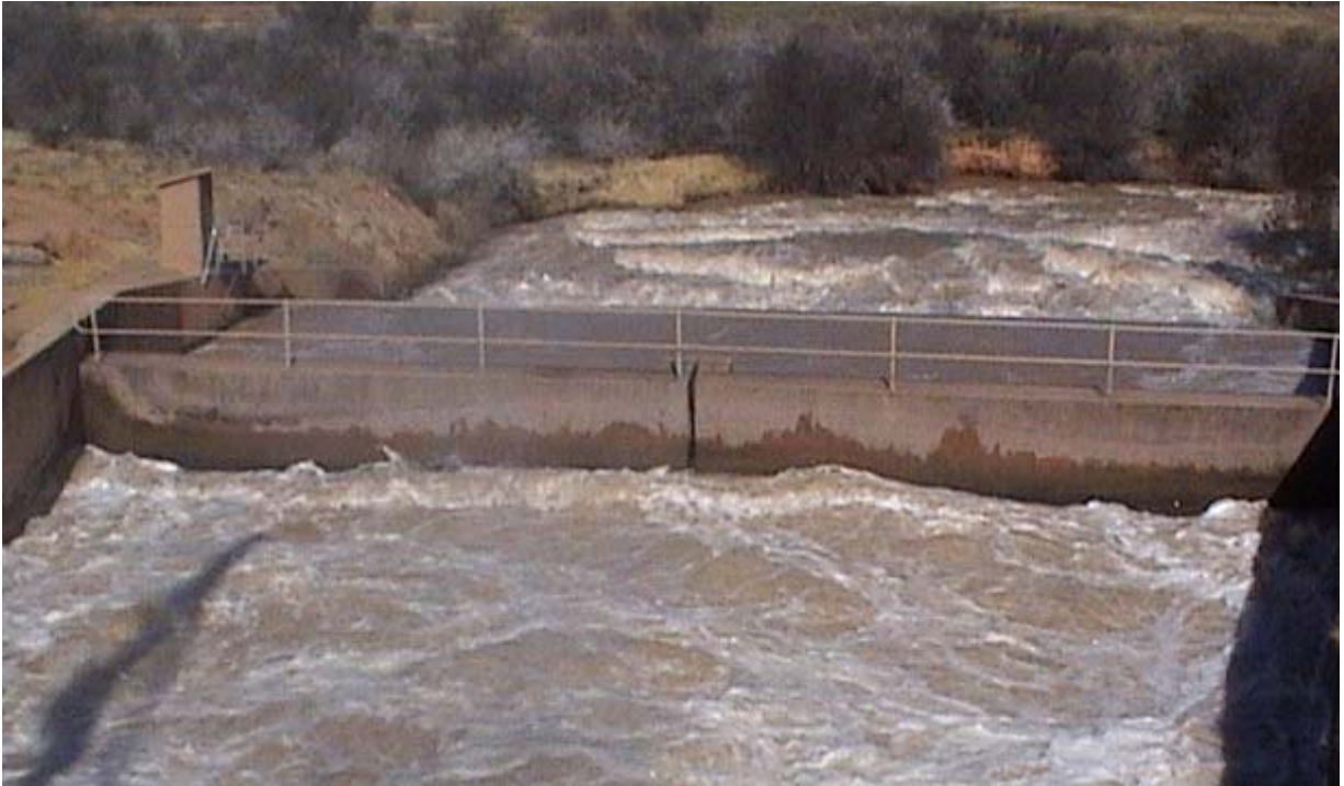
Figure 5.10-3: The Energy Dissipater and Flow Gauging Station below the Outlet Gates of Grassridge Dam
