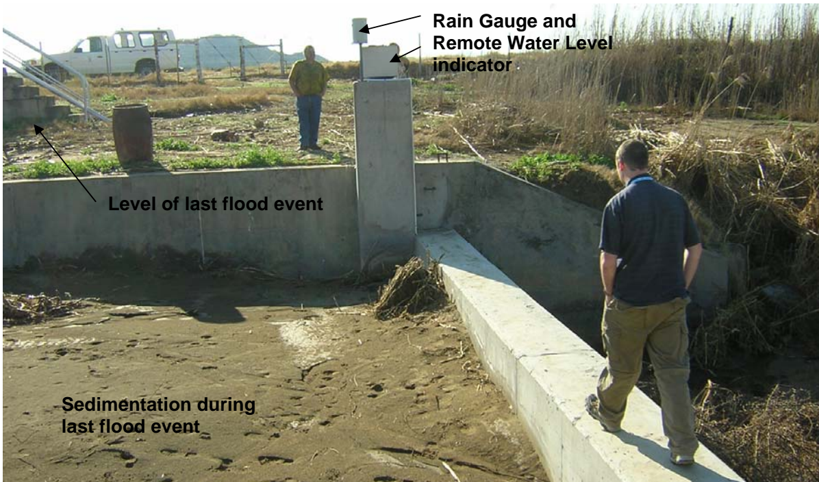
Figure 7.1-6: Waaikraal Weir, showing the Side Walls and the Last Flood Level at the Weir
