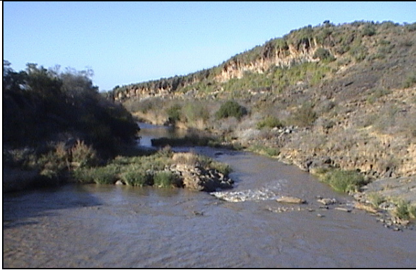
Figure A-26: Hermanuskraal Weir
