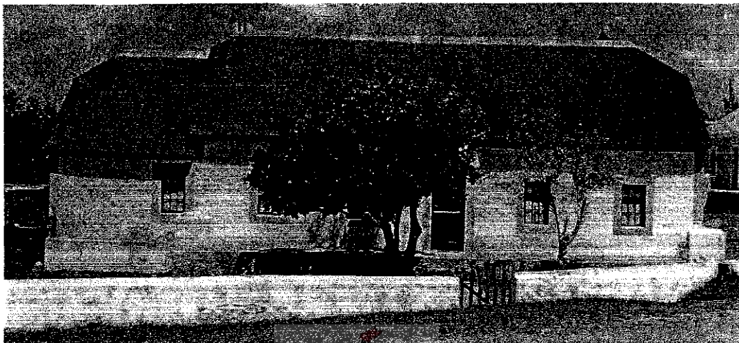
Figure 94: This building is a synthesis of the kerkwerf architecture and the cottage style, in the rustication detail having been applied to a slightly enlarged version of cottage no 3 (figure 186) (L van der Hoven 1999).
