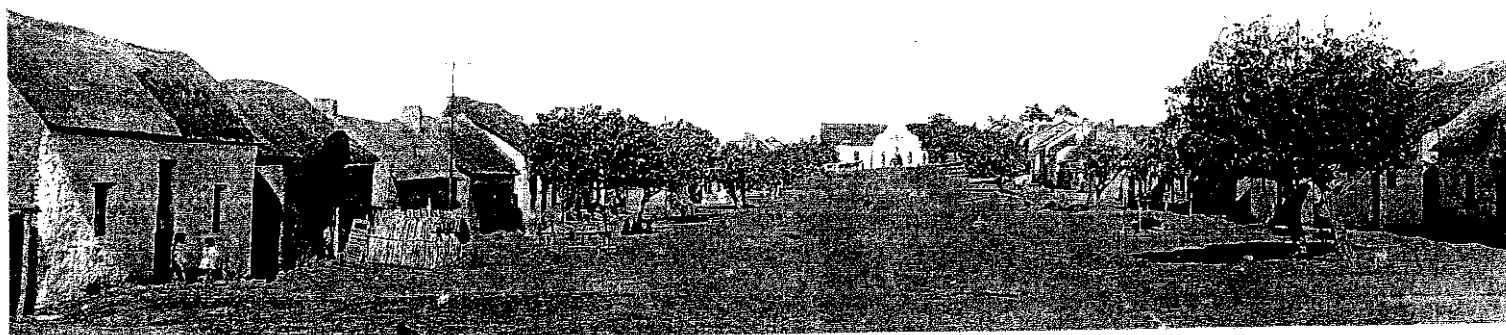
Figure 181: Kerk Street seen from a greater distance to the church (Cape Archives Depot:R512).
