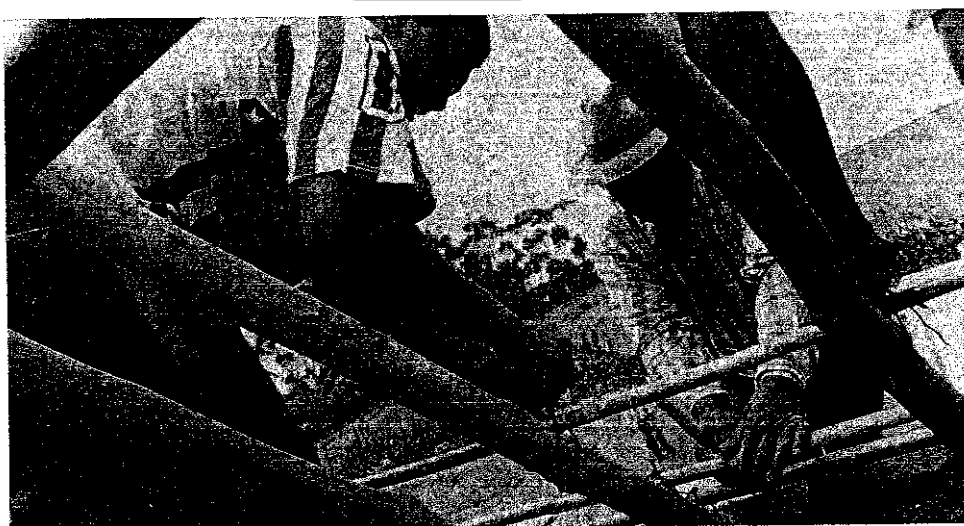
Figure 264: New spaansriet supports are placed horizontally parallel and measured by Mr Neels Afrika before being tied into place with tarred string (L van der Hoven 1997).
