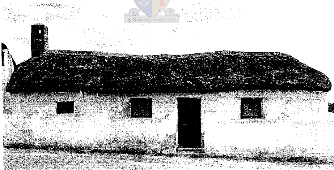
Figure 272: The thatch of an east- west facing cottage in Sand Street is worn thin with age and has some plants growing in it. The reason it has endured so many years is because it is in the full sun (L van der Hoven 2001).
