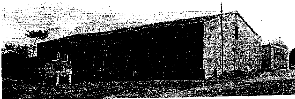
Figure 170: Old Bloemenhuis just before it was knocked down, with the new shed to the south already completed (L van der Hoven 1998).
