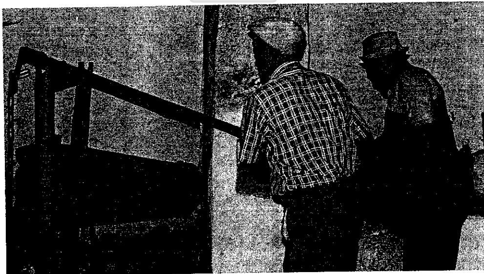
Figure 153: Christie Cloete rhythmically operates the bellows while Mattheus Daniels tends the fire where the hoop of the wagon-wheel will be heated (H Wessels 1998).
