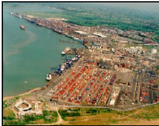
Figure 12: Port of Felixstowe, UK (Courtesy of the Port of Felixstowe)
