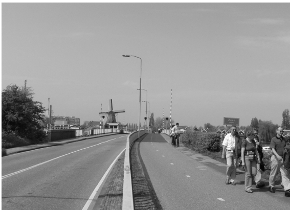
Figure 7a: Separate traffic lanes for automobiles, bicycles and pedestrians . Location: Zaanseskans, The Netherlands Source: A Theart, April 2005
