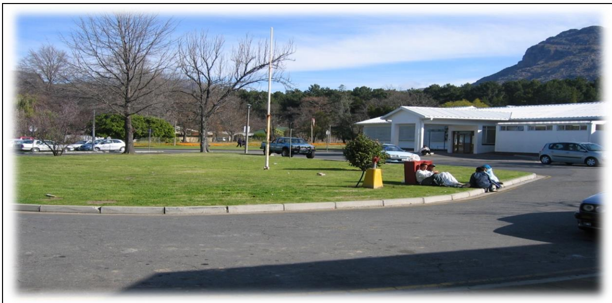
Figure 1: Ceres District Hospital
