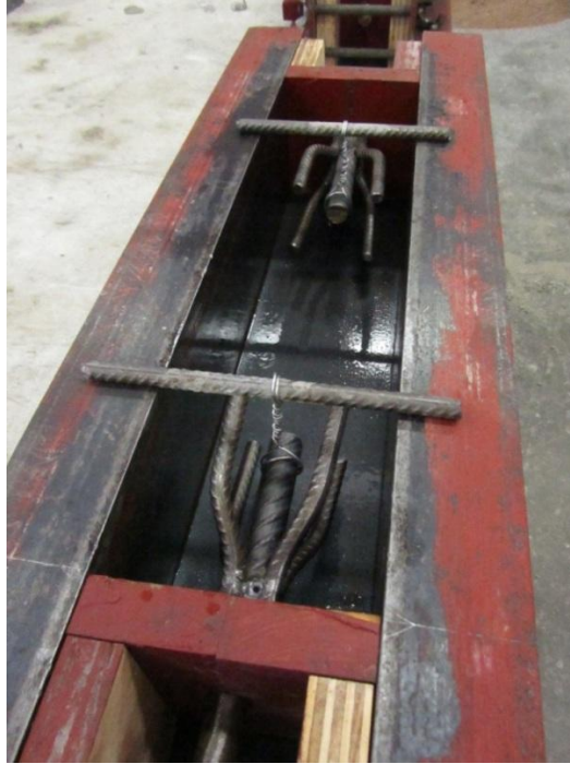
Figure 21 Beam mould ready for casting.
