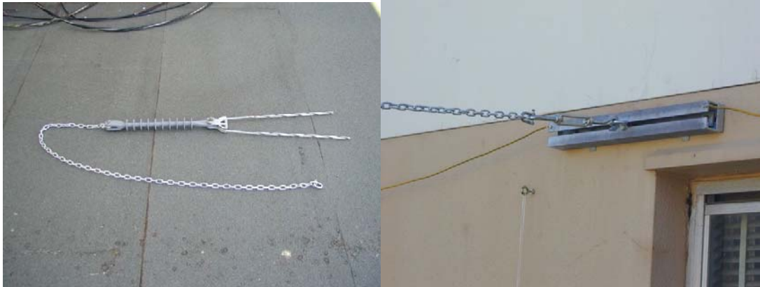
Figure 8.7: Chain and insulator used to connect HV cable to bracket.
