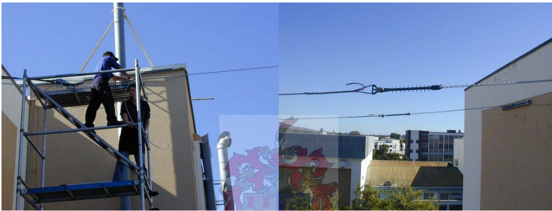
Figure 8.8: (a) Adjustment of cables and (b) cables after suspension.
