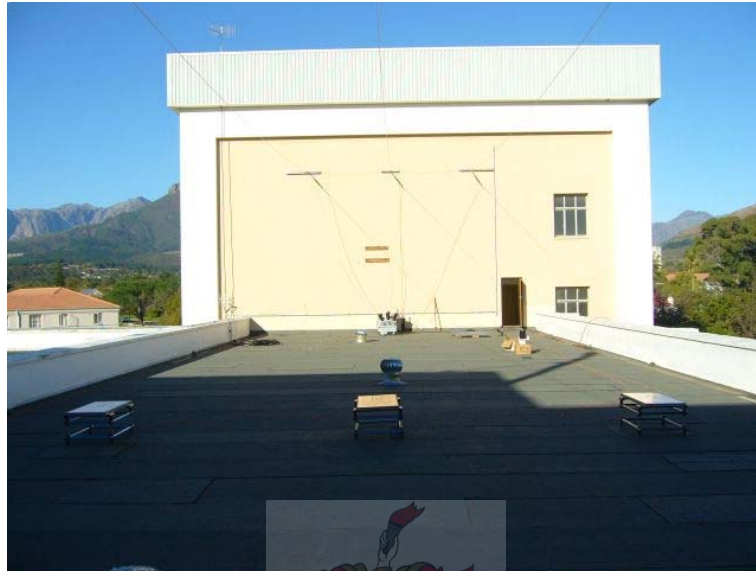
Figure 8.17: HV Test facility with the three sensors centralised underneath the conductors.
