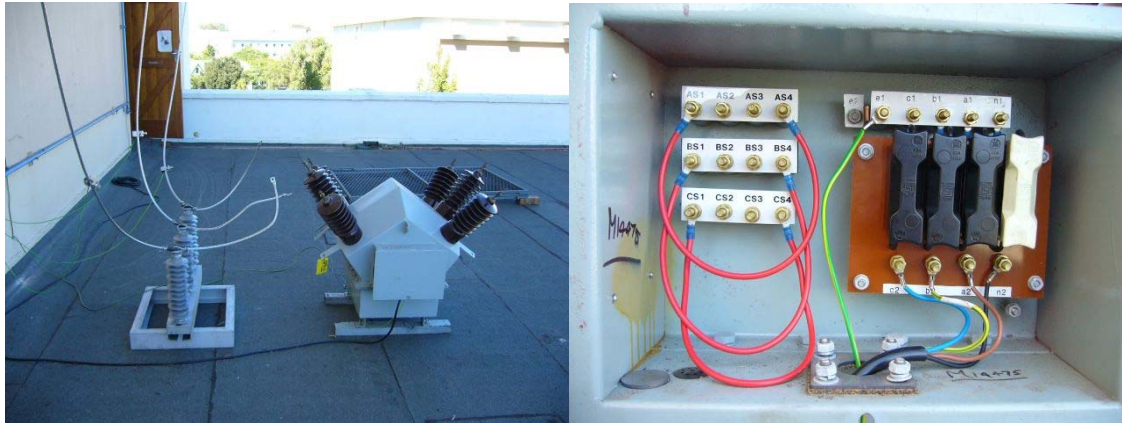
Figure 8.9: (a) Three-phase transformer used at test facility and (b) wiring of the transformer.
