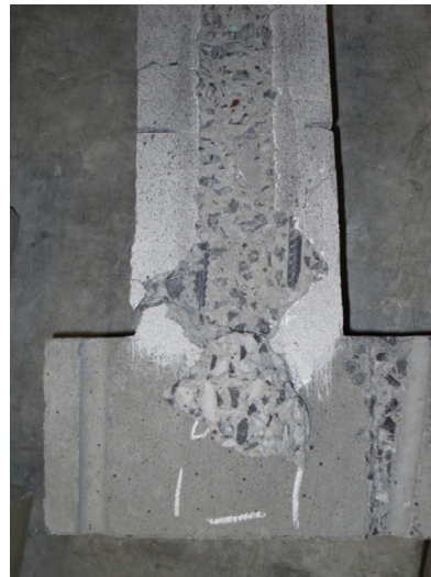
b.) Concrete cover separation
