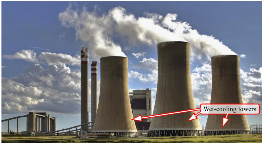
Figure 1.1: Cooling towers (Source: carbon-power [Sat])
