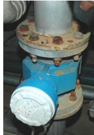
Figure 3.8: Photo of electromagnetic flow meter installed in water supply line
