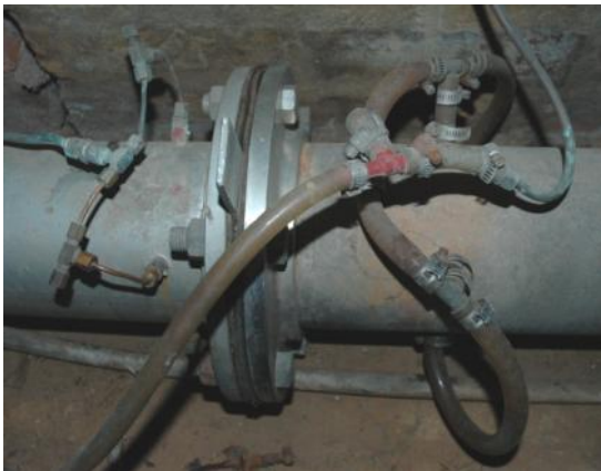
(a) Orifice plate in water supply line
