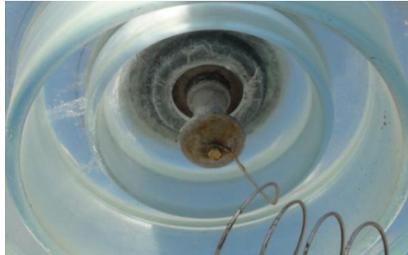
Figure E-95: The first instance of material erosion on the bottom of glass disc around the pin (Week 6)
