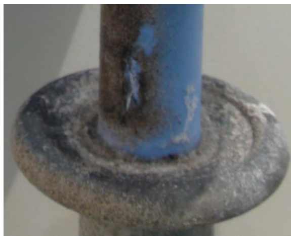
Figure E-74: The first sign of material erosion on the sheath interfacing with the live end-fitting in the southward direction (Week 5)
