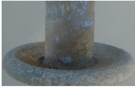
Figure E-89: Rust deposit on the sheath interfacing with the live end-fitting in the westward direction (Week 18)
