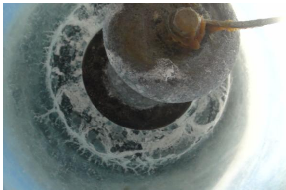
Figure 5-38: Material erosion on the bottom of Glass disc 42 DC- around the pin, week 16
