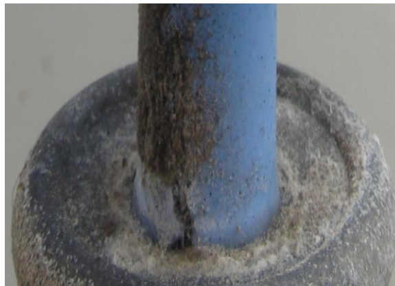
Figure E-83: Dark burns on pollution on the sheath interfacing with the live end-fitting (Week 5)
