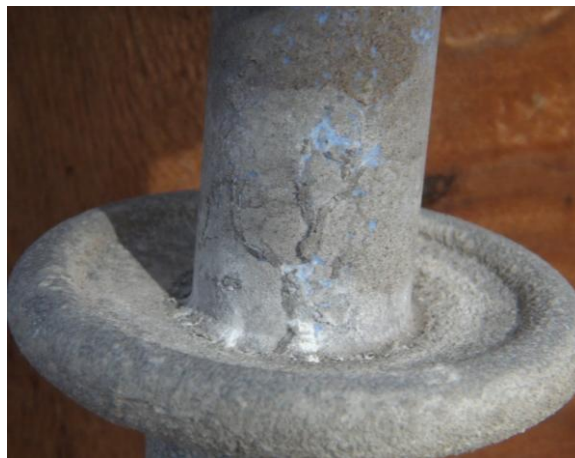
Figure E-90: Material erosion on the sheath interfacing with the ground end-fitting (Week 16)
