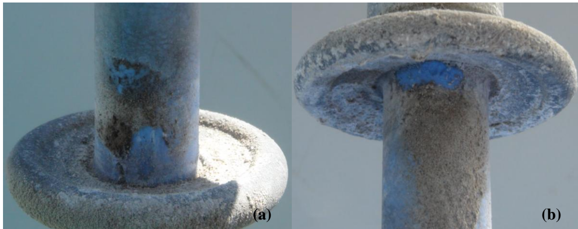
Figure E-85: The first signs of erosion on the sheaths interfacing with both the (a) live and (b) ground end-fittings in the southward direction (week 8)
