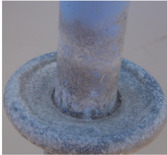
Figure E-41: Material erosion on the sheath interfacing the the live end-fitting in the westward direction (Week 16)
