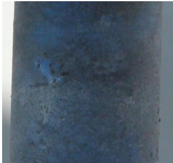
Figure E-78: Material erosion on the sheath interfacing with the live end-fitting (Week 11)
