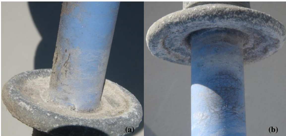
Figure E-30: Material erosion on the sheath interfacing with the live end-fitting and (b) light crazing on the sheath interfacing with the ground end-fitting (Week 9)
