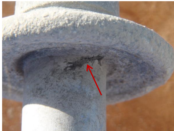
Figure E-39: Material erosion on the sheath interfacing with the ground end-fitting (Week 22)
