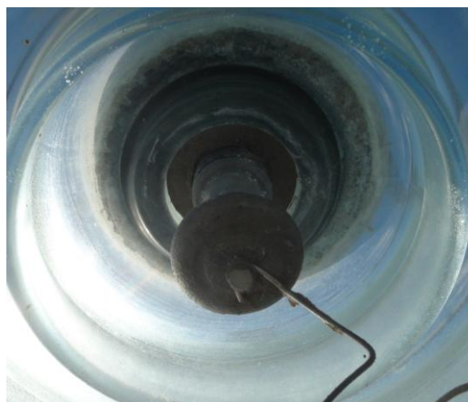
Figure E-96: Traces of dryband activity on the bottom of glass disc around the pin (Week 13)
