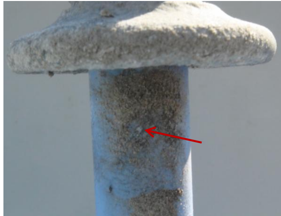
Figure E-37: Material erosion on the sheath interfacing with the ground end-fitting along the heavy pollution deposit on HTV-SR 84 DC- (Week 10)
