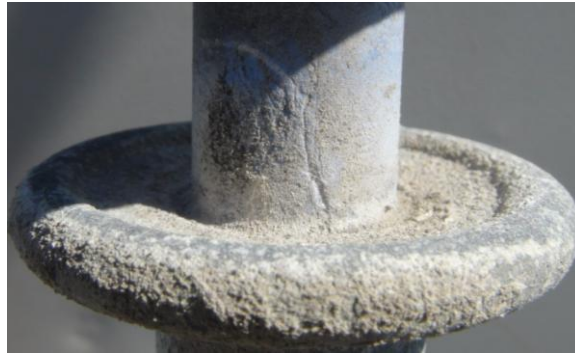
Figure E-86: Material erosion on the sheath interfacing with the live end-fitting (week 13)
