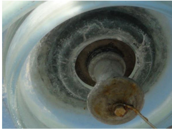
Figure E-98: Material erosion on the bottom of glass disc around the pin (Week 10)
