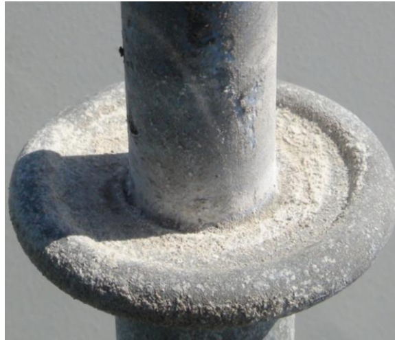
Figure E-53: Material erosion on the sheath interfacing with the live end-fitting (Week 10)
