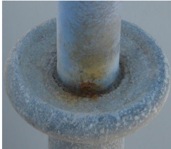
Figure E-58: Rust patches on the sheath interfacing with the live end-fitting (Week 18)
