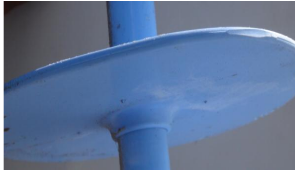
Figure E-27: Traces of dryband activity visible on the shed bottom of HTV-SR 84 DC+ (Week 3)
