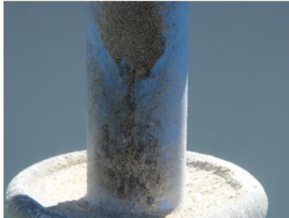
Figure E-62: Material erosion on the sheath interfacing with the live end-fitting in the southward direction (Week 9)
