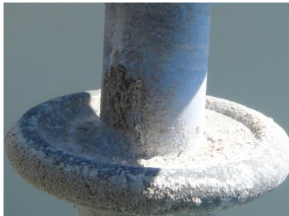
Figure E-84: The first sign of material erosion on the sheath interfacing with the live end-fitting in the southward direction (Week 9)
