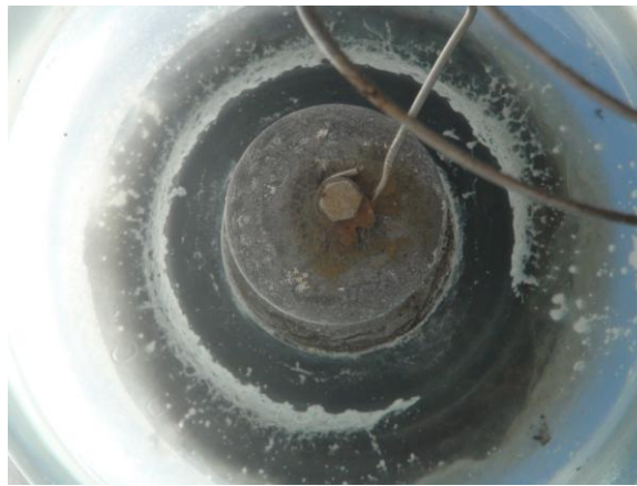
Figure E-97: Material erosion on the bottom of glass disc around the pin (Week 11)
