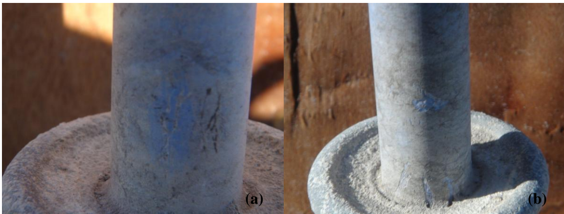
Figure 5-35: Two instances of material erosion on the sheath interfacing with the live end-fitting in the (a) southward direction and (b) northward direction, week 22
