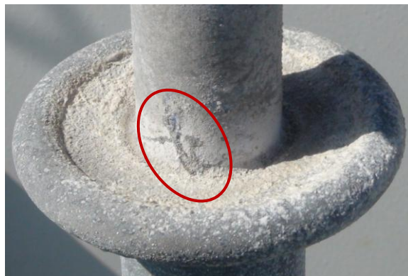
Figure E-67: Material erosion observed on the sheath interfacing with the live end-fitting (Week 10)
