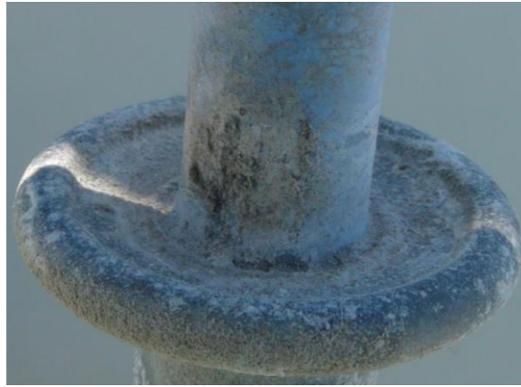
Figure E-75: Erosion on the sheath interfacing with the live end-fitting in the southward direction (Week 9)
