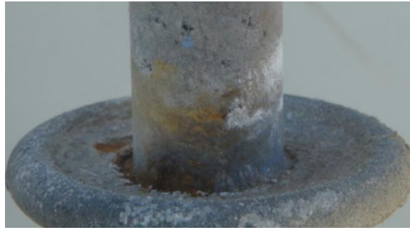
Figure E-87: Rust deposit on the sheath interfacing with the live end-fitting in the westward direction (Week 11)
