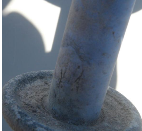
Figure E-34: Material erosion on the sheath interfacing with the live end-fitting of HTV-SR 84 AC (Week 13)
