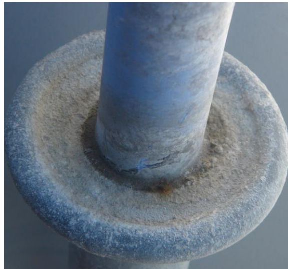
Figure E-40: Material erosion on the sheath interfacing with the live end-fitting in the southward direction (Week 18)
