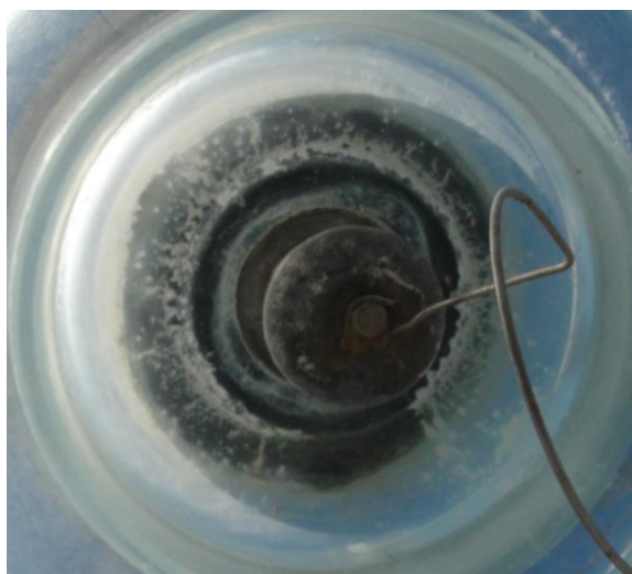
Figure 5-37: Material erosion on the bottom of Glass disc 42 DC+ around the pin, week 18
