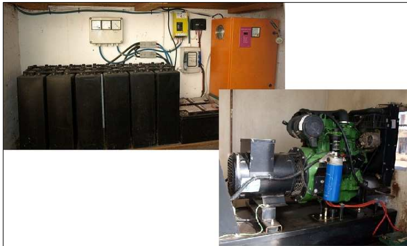
Figure 4-3: Battery bank and generator
