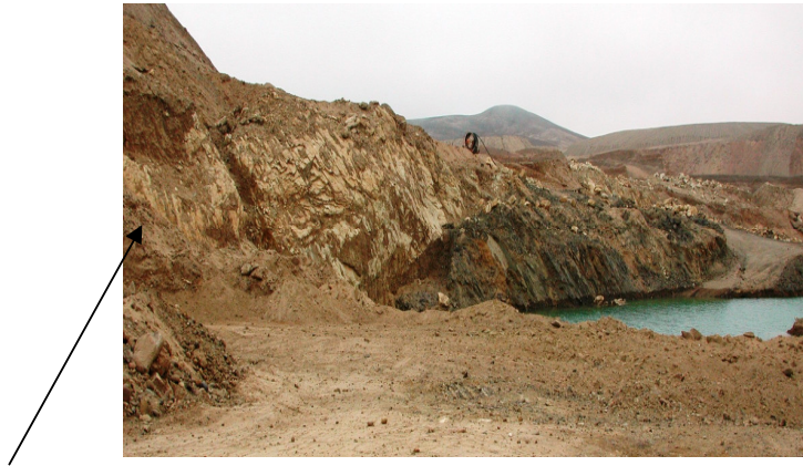
Fig. 2.14 Aplite dyke with downstream scour, Koeskop Mining Area, Baken Mine. (Camera facing upstream, viewer standing on back-filled portion of deep scour)
