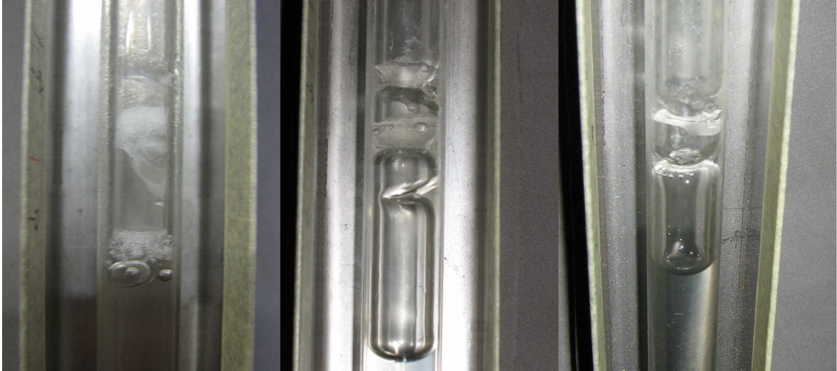
Figure 5.11: Ice in the evaporator sight glass
