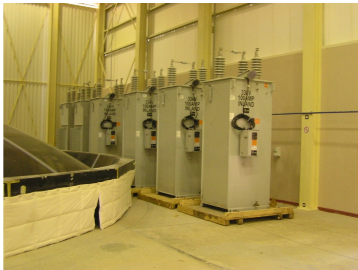
Figure 5-9: Voltage Regulators in Storage
