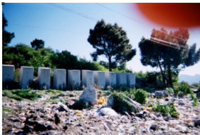
Figure 4.12: 'This the toilets that the community is use.' (Participant quote)
