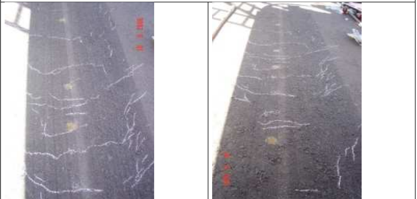
Plans views of test sections, with surface cracks marked
