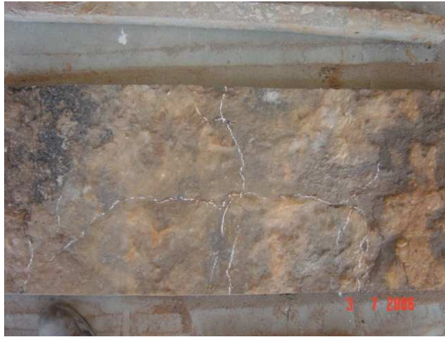
Figure 3.17c: View of underside of HMA extracted from full scale test section 4 after 340 000 load repetitions for diagnostic investigation showing marked positions of cracks
