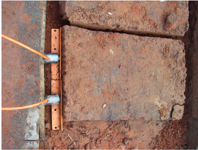
Figure 3.19c: Shifting of CTB block with hydraulic jack to prevent formation of non-traffic related fractures
