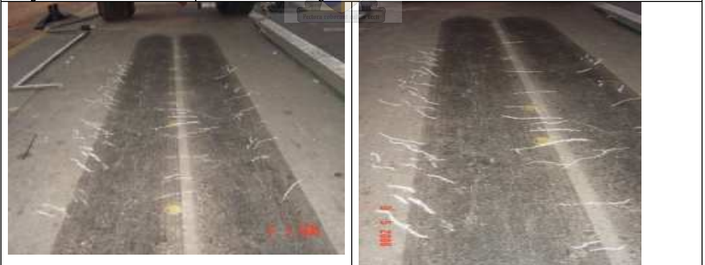
Diagonal shear crack development on outer edges of wheeltrack
