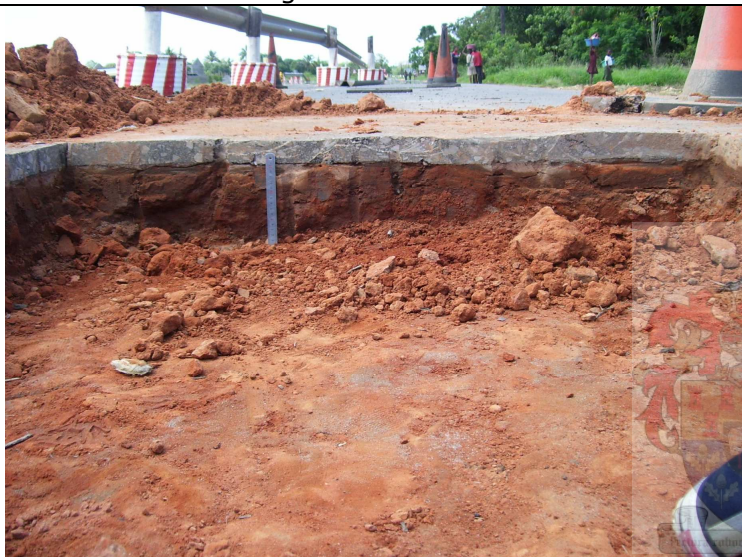
Pictorial views of diagnostic trench after excavation.
