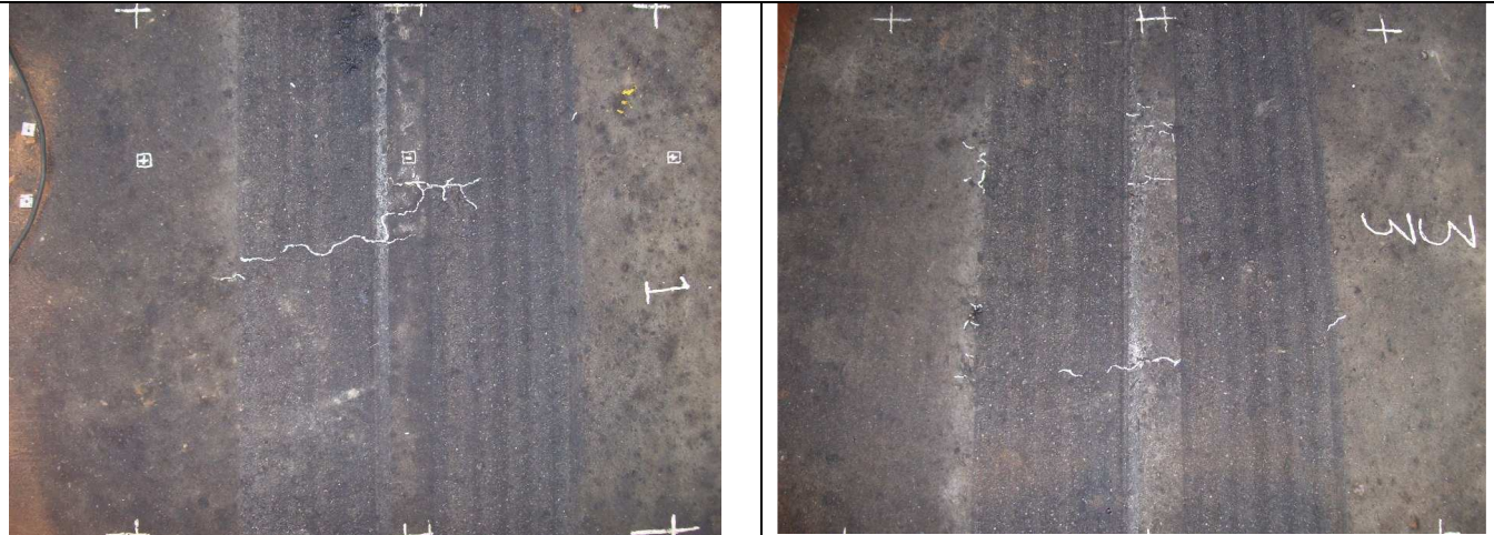
Plan views of test section with crack marked in white
