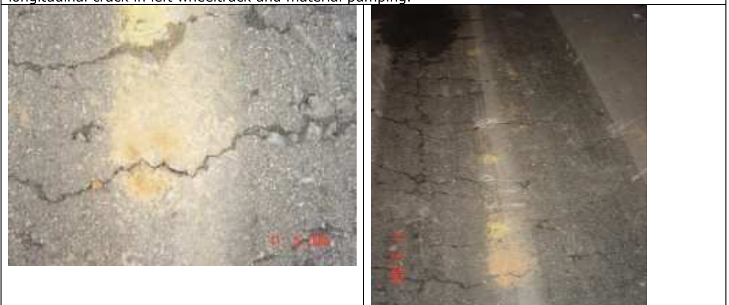
Surface cracking pattern after wet trafficking, note completed transverse cracks, formation of longitudinal crack in left wheeltrack and material pumping.
