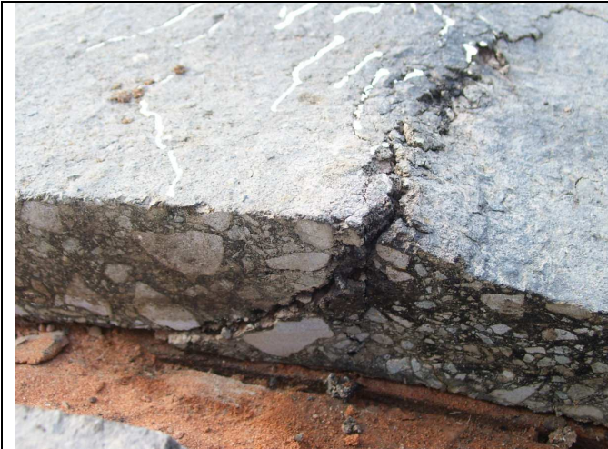
Close ups of HMA vertical shear
