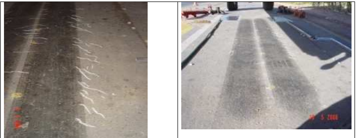
Diagonal shear crack development on outer edges of wheeltrack
