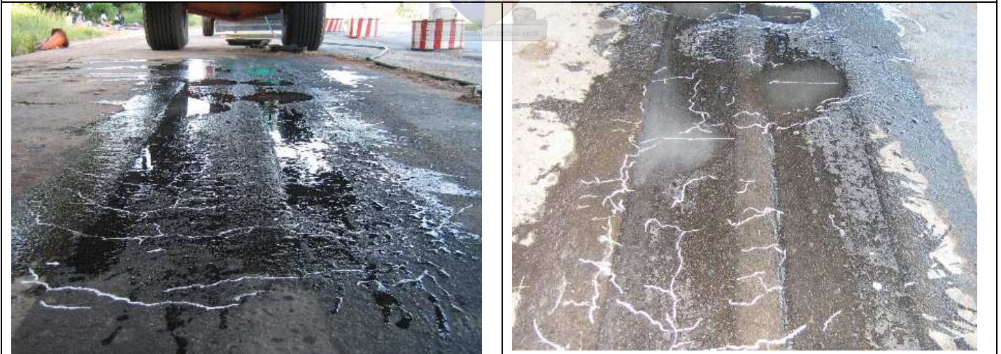
Pictorial overviews of test section with cracks marked in white.
