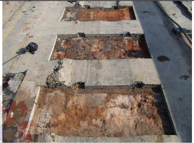
Underside of HMA mat after removal of test pit 3. Pictorial overview of all test pits with HMA removed.
