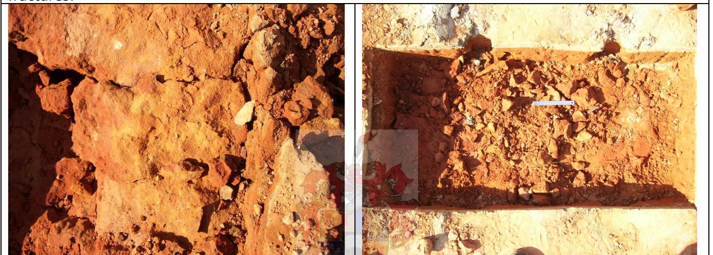
Fractured CTB and plan view of test pit after removal of CTB fractures.
