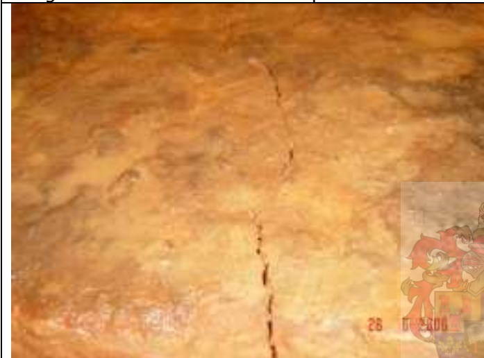
Longitudinal crack taken from the top side of the CTB block
