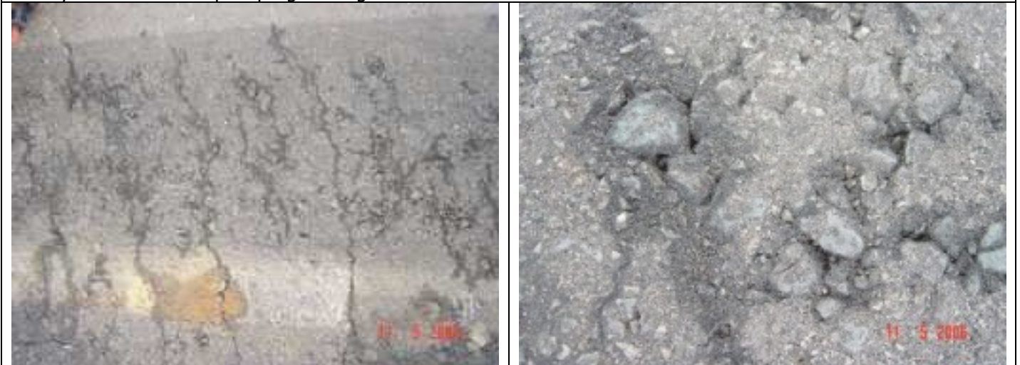
Surface crack pattern and texture after wet trafficking
