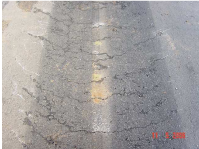
(c) Continuous transverse cracks and longitudinal crack formation after 320 000 60 kN load applications - Section 4
