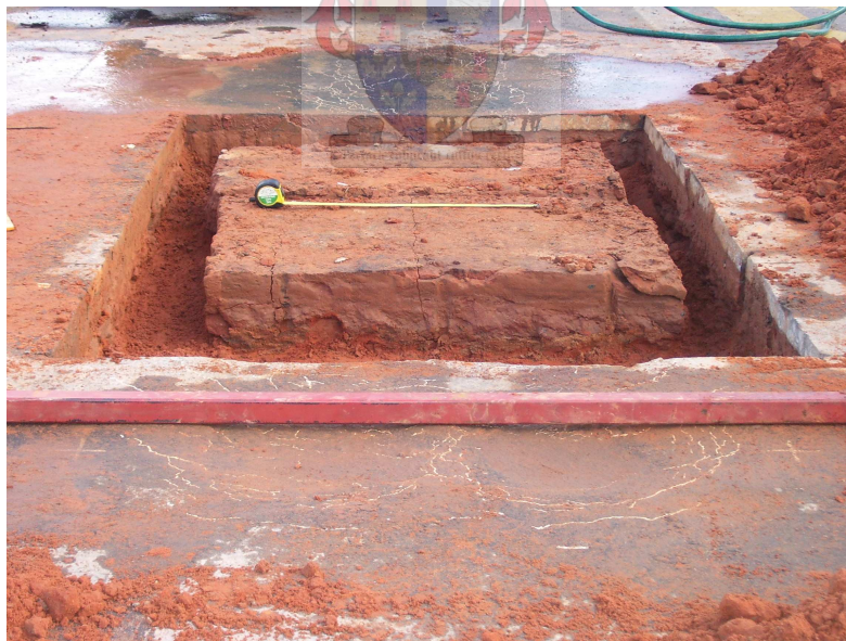
Figure 3.19b: CTB block ready for removal all surrounding CTB material
