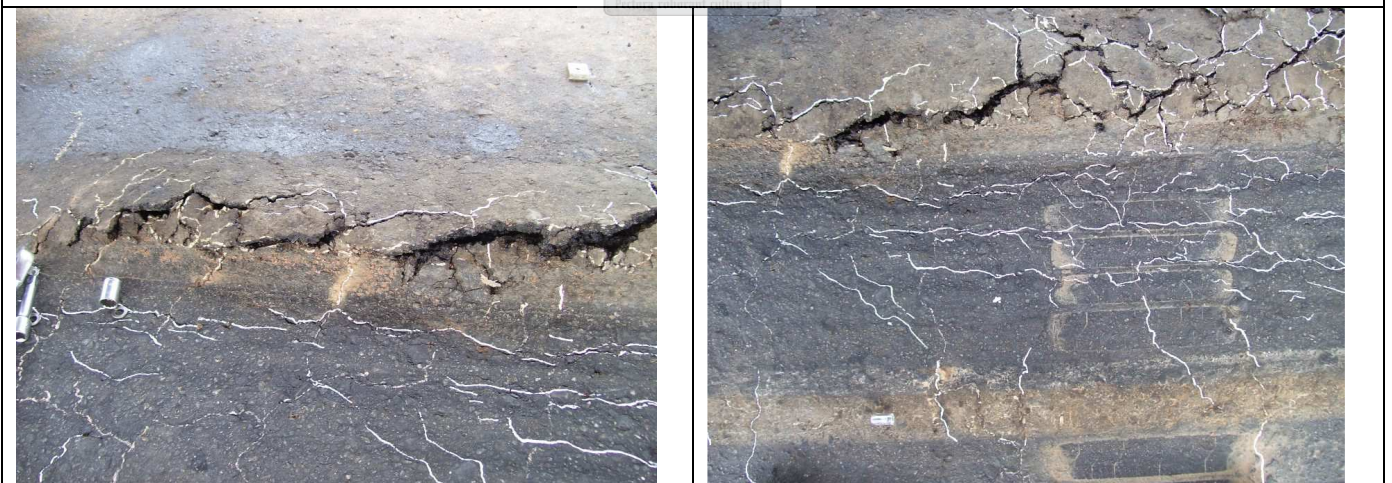
HMA heaving and cracking on the side of the wheeltrack. Note extensive crack pattern in wheeltrack
