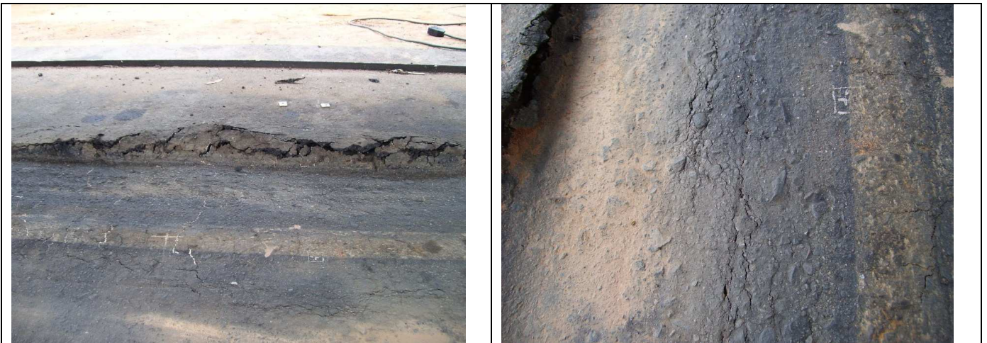
Heaved HMA on side of wheeltrack
