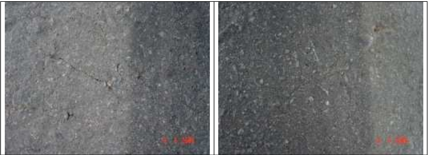
Surface crack initiation after 250 000 60 kN load applications
