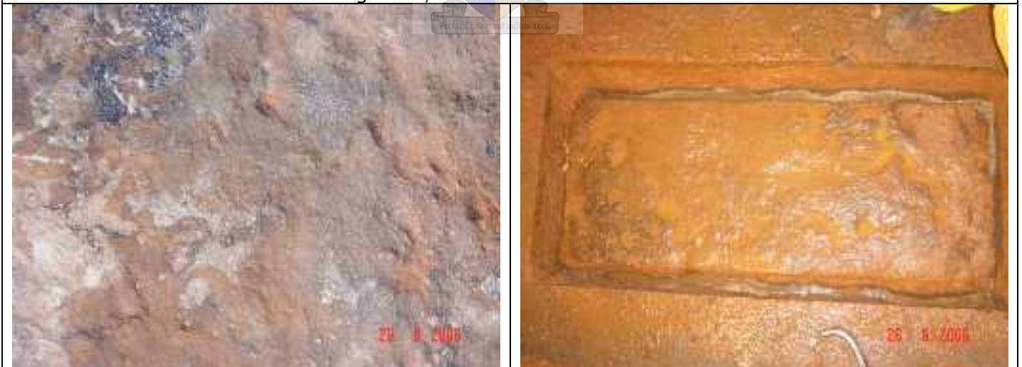
Underside of removed HMA slab and top view of CTB slab after removal of enclosed material
