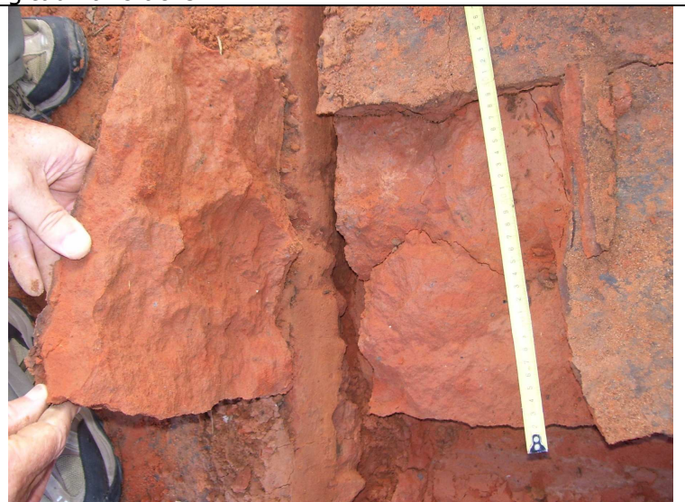
Pictorial overview of blocks and extraction of top part of CTB. Note mid layer shear plane intersecting with longitudinal and transverse cracks
