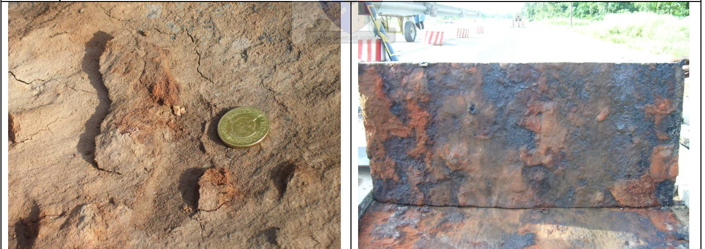
Close up of CTB surface after removal of HAM. Note smoothed surface texture. Underside of HMA mat removed from test pit 2.
