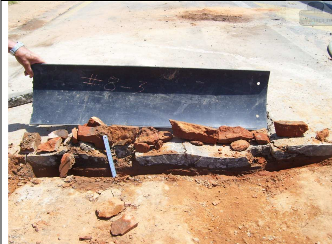
Removal of CTB fractures.
