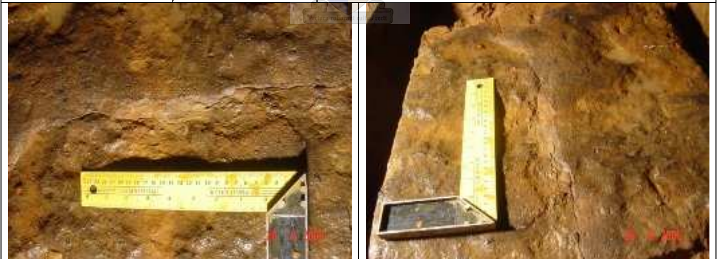
Transverse crack in CTB, views taken from top of CTB block
