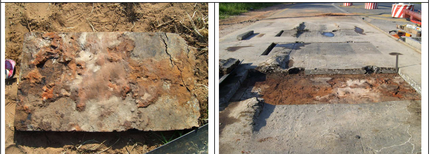
Underside of removed HMA mat. Note smoothed interface surface due to shear fatigue.
