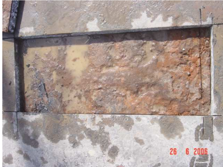
Figure 3.19a: Removed HMA after dual box cut by diamond blade grinder
