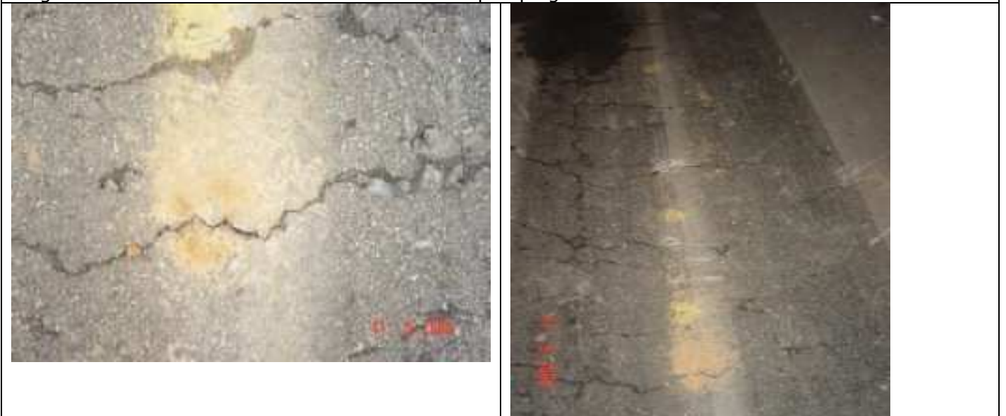
Surface cracking pattern after wet trafficking, note completed transverse cracks, formation of longitudinal crack in left wheeltrack and material pumping.
