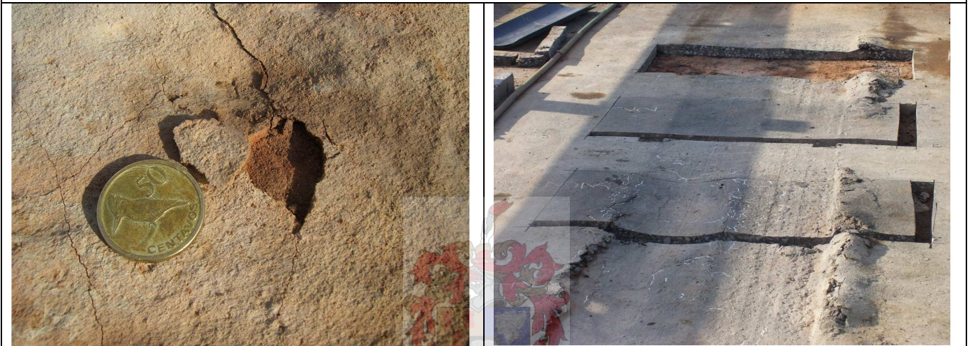
Close up of CTB surface after removal of HAM. Note smoothed surface texture.
