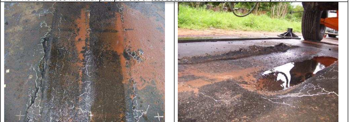
Plan and pictorial views of base material pumped out of test section. Note extensive crack patterns
