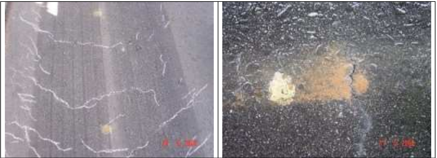
Transverse crack completed and material pumping
