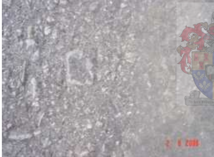
HMA surface texture. Note stripping of asphalt
