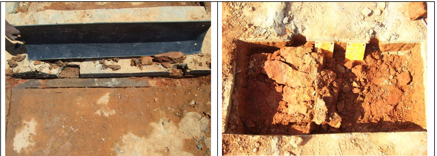
Removal of CTB fractures. Plan view of test pit during removal of CTB fractures note the size of the fractures.
