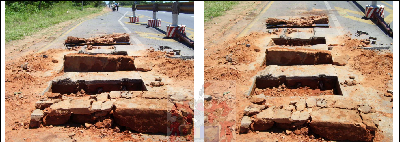
After completion of diagnostic trenching note reconstituted CTB slab in front of picture.
