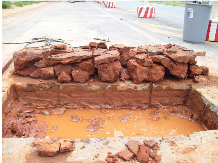
(a) Front view - note horizontal shear plane and longitudinal cracks
