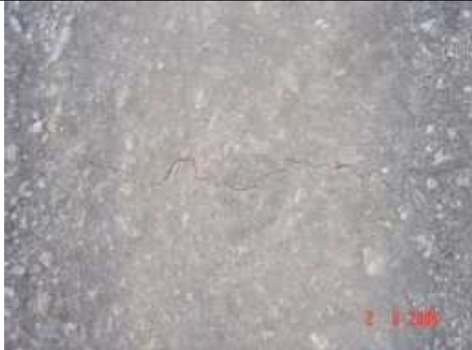
Transverse crack formation
