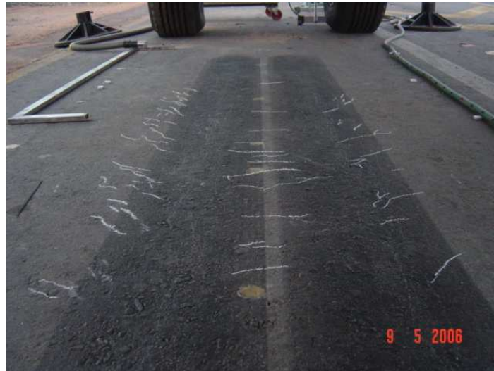
(a) Transverse shear crack initiation at 270 000 60 kN load applications - Section 4
