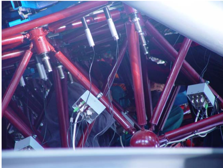
Figure 3.3: SALT mirror support truss: Close-up of struts and nodes (SALT Foundation, 2011)
