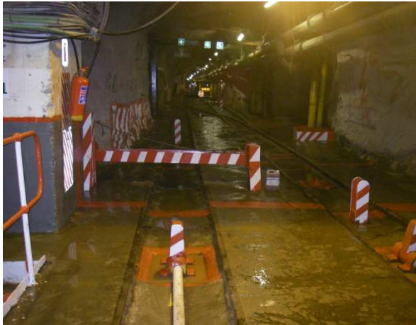
Figure 16a: A typical underground walkway
