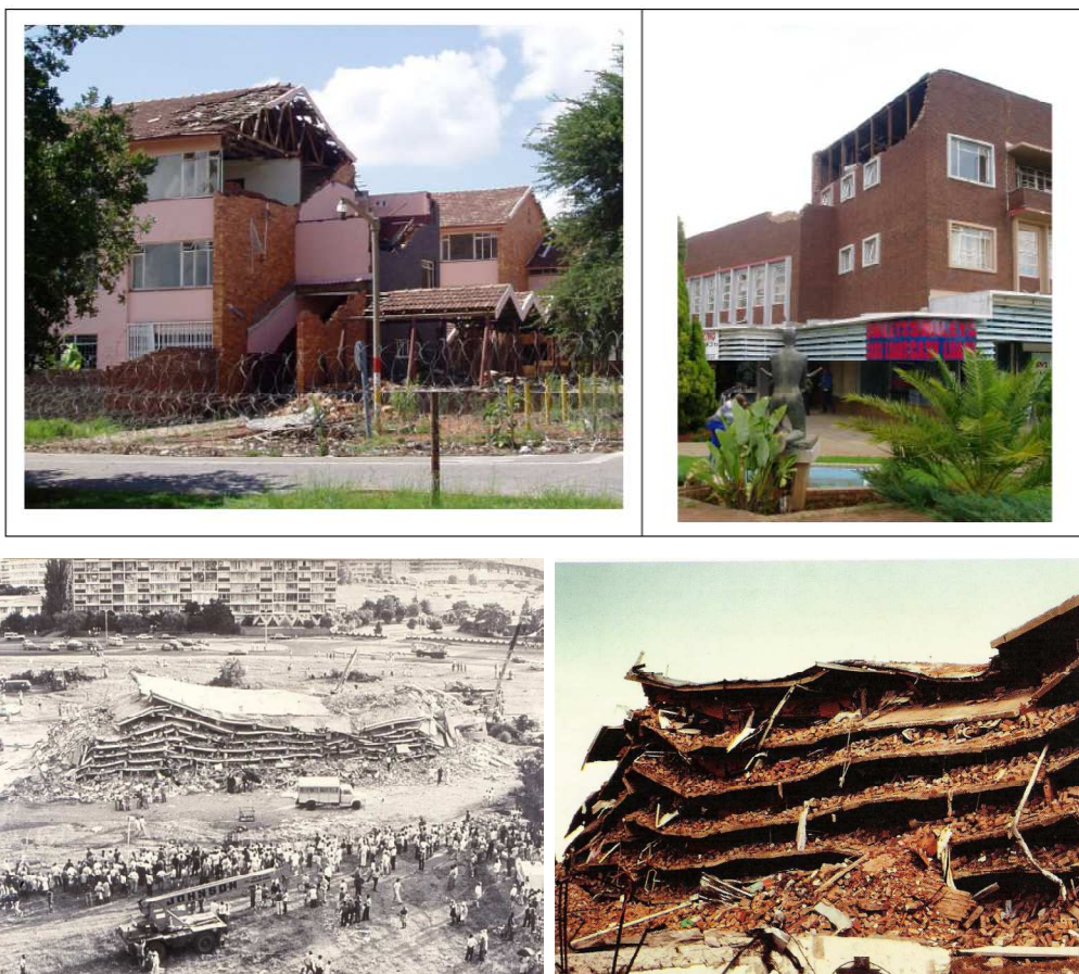
Figure 10: Damage to buildings as a result of mining related earthquakes in Stilfontein and Welkom South Africa Source: Goldbach, 2010.
