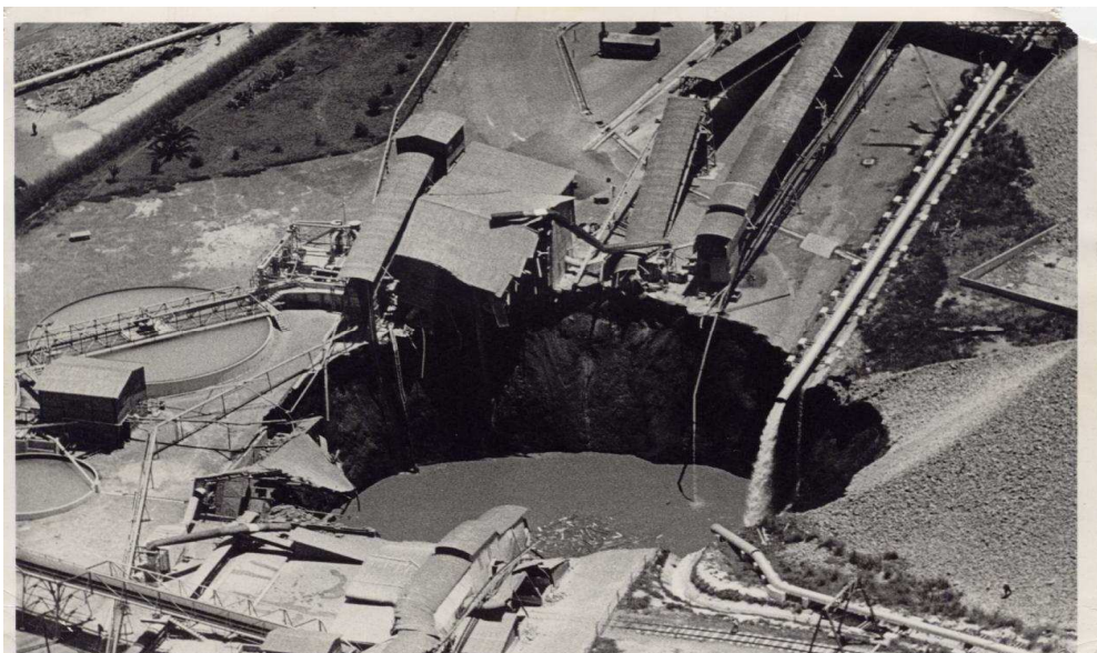
Figure 14: A sinkhole that developed at Gold Au property in 1962
