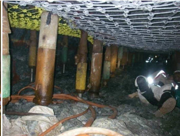
Figure 16b: A typical Stopping area
