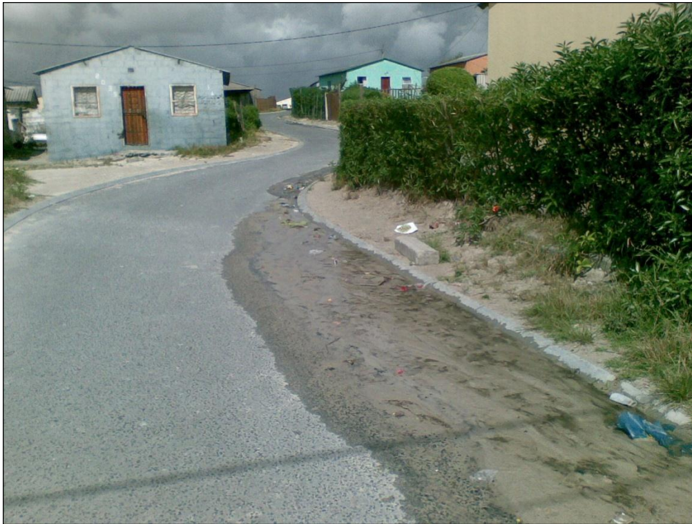
Figure 27: Wastewater running down a street in Driftsands. This water carries large amounts of sand into the storm water system causing further blockage
