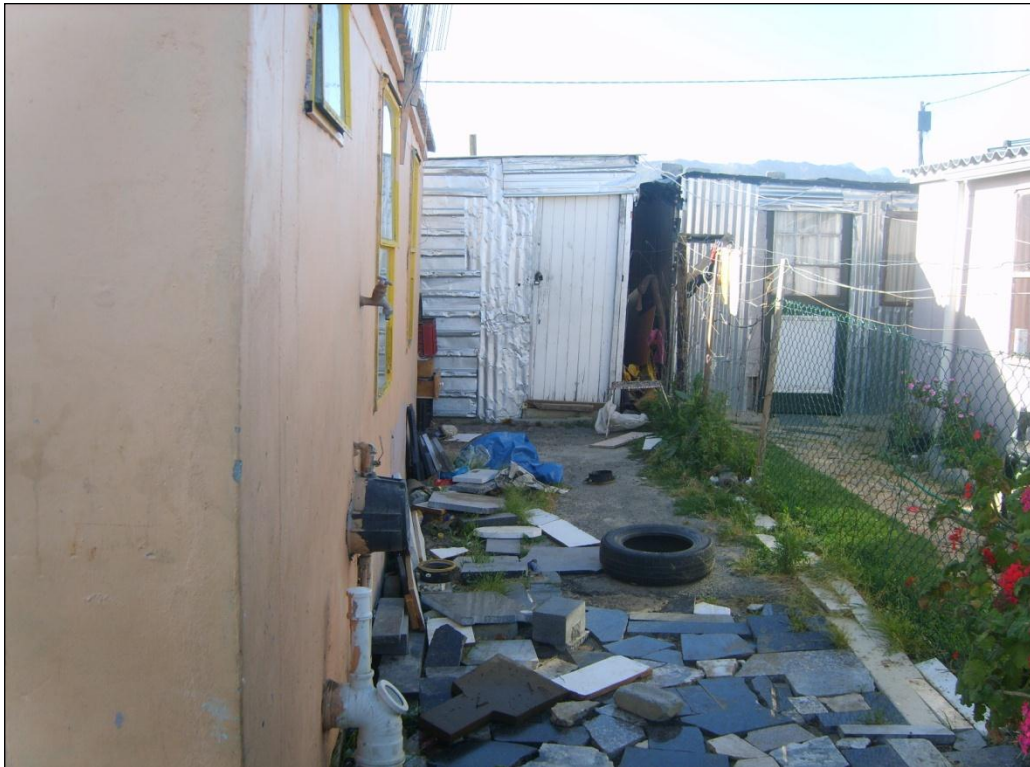
Figure 5: Virtually no space between shacks on adjacent plots – which are against municipal building codes. Note the tap on the left hand side wall with no drain to receive dirty water. Solid waste distributed on premises on the left
