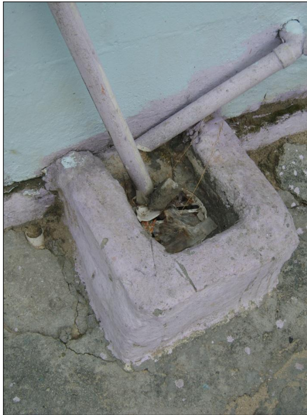
Figure 23: An example of a blocked outside drain in Tafelsig
