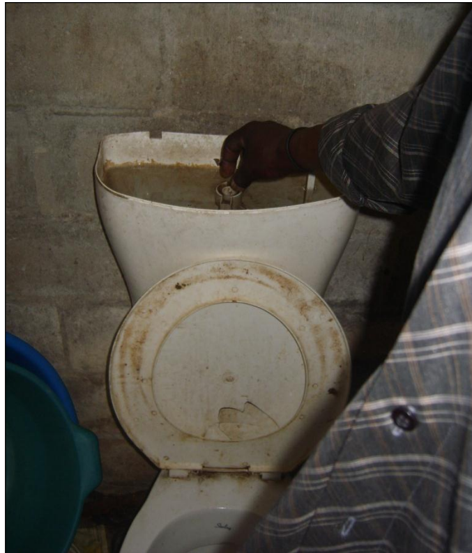
Figure 15: Flushing mechanism on this toilet is broken. Users flush toilet by manually manipulating the mechanism inside the system. Note that the toilet is dirty
