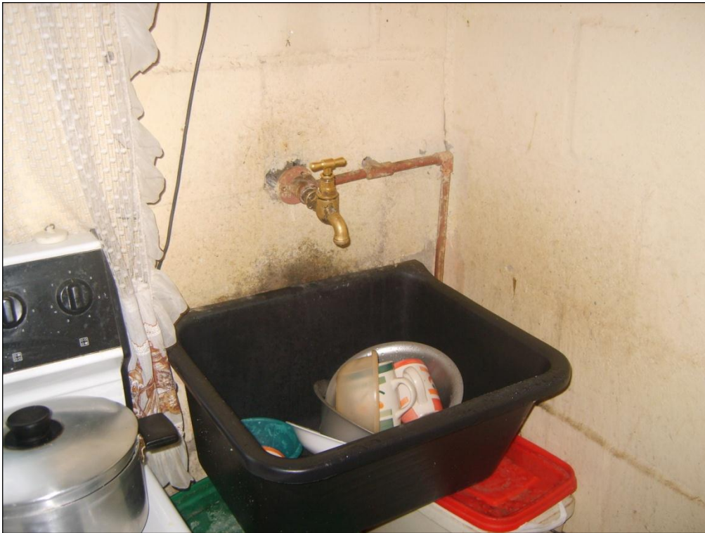
Figure 19: An example of a kitchen area in Greenfields. Note the rudimentary facilities and dirty wall. This is the only working tap in the main house
