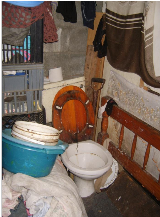
Figure 17: Toilet used as storage area in Tafelsig
