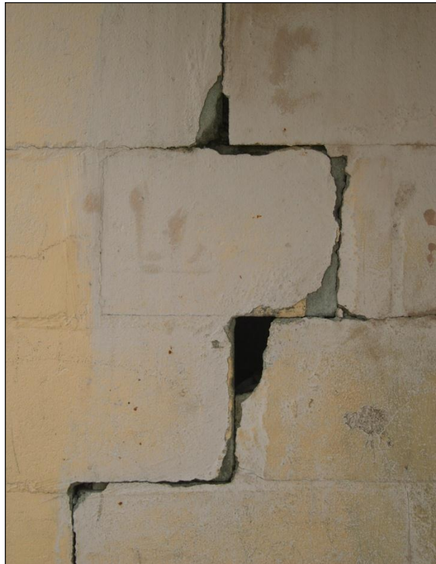
Figure 11: An example of structural damage – seriously cracked wall of main house
