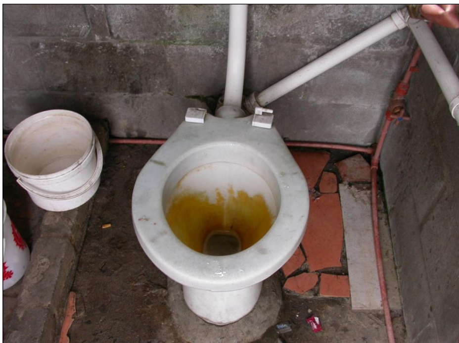
Figure 12: An example of a dirty toilet and wet walls in Driftsands
