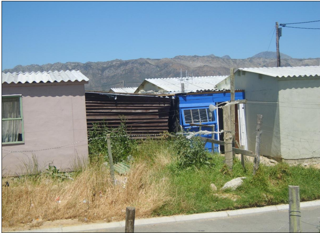
Figure 3: Adjoining shacks in the Greenfields settlement obscuring municipal reticulation systems
