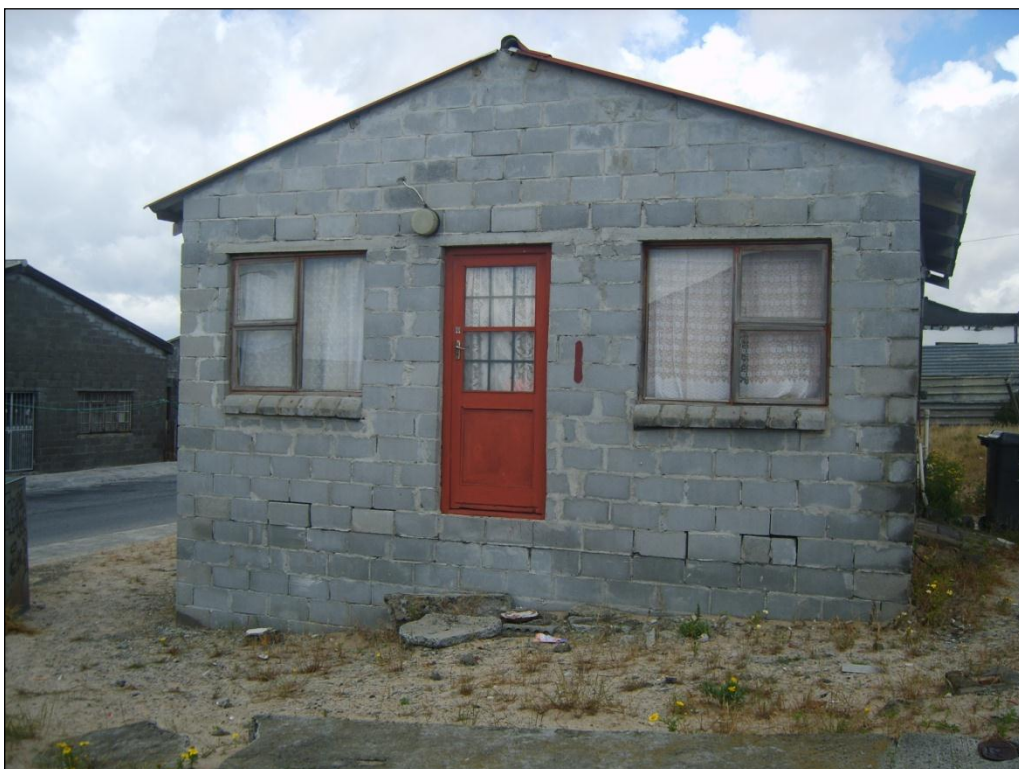
Figure 8: Design of the main house is inappropriate for the terrain. Access to this house difficult is for the young, the aged and the physically challenged
