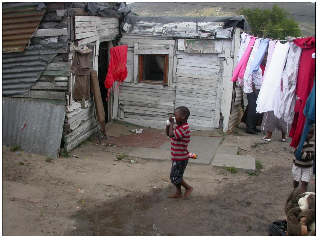
Figure 4: Makeshift shack structure in Tafelsig. Note the flimsy building materials
