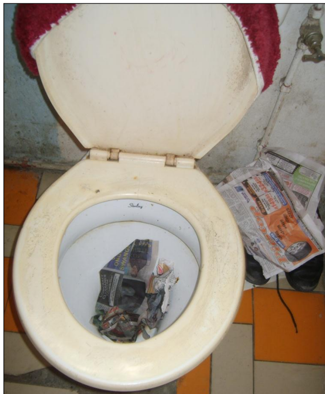
Figure 16: An example of a blocked toilet in Masipumelela. Note the newspaper used as wipes
