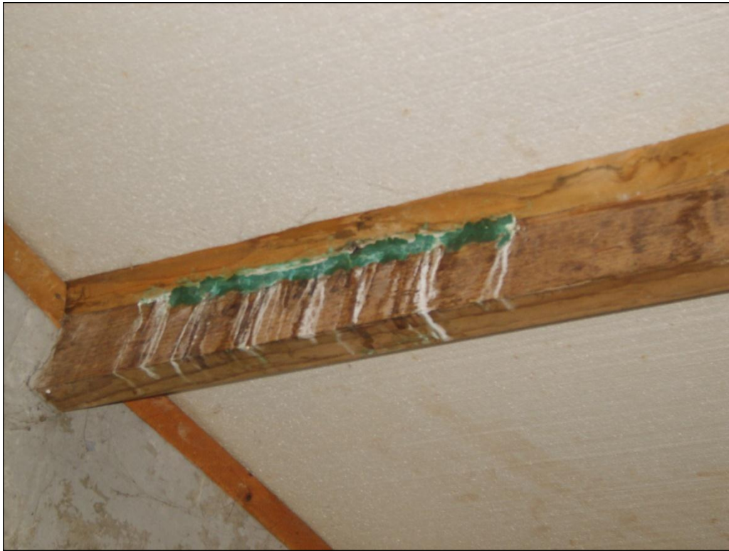
Figure 9: Leaking roof structure inappropriately fixed with soft soap
