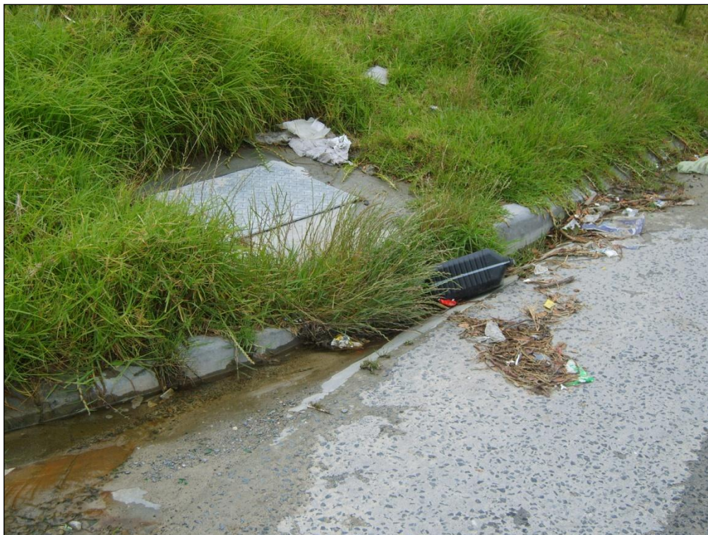
Figure 26: Faecally polluted drainage water running into storm water inlet in Masipumelela. Therefore the abundant growth of grass due to the fertilizer effect of polluted water. This growth also invades the storm water system causing further blockage
