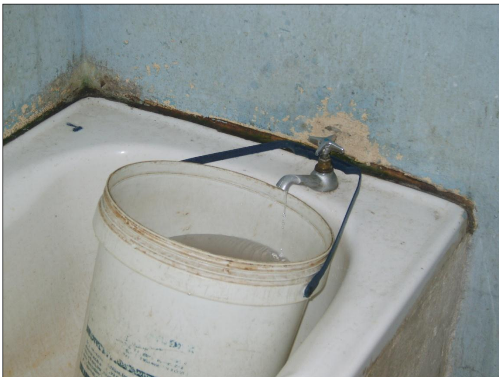
Figure 20: An example of the bathroom area in the Tafelsig settlement. There is only cold water provided. This unrepaired tap leaks permanently
