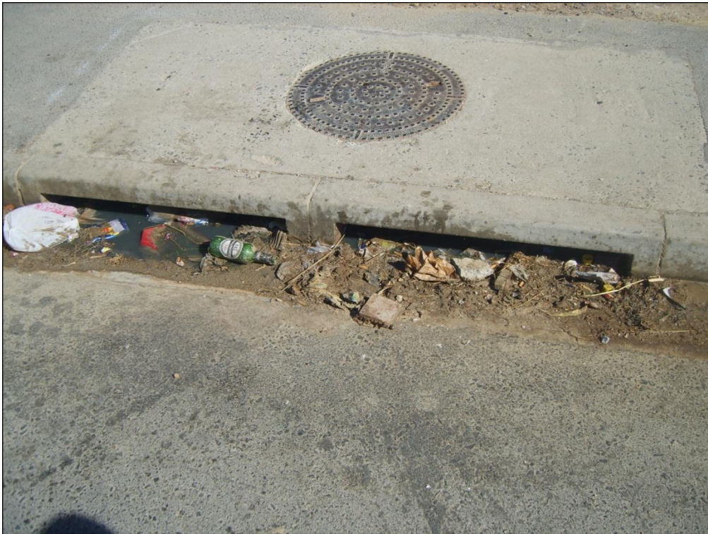
Figure 25: Solid waste blocking the storm water inlet on street causing subsequent flooding during rain storms in Tafelsig
