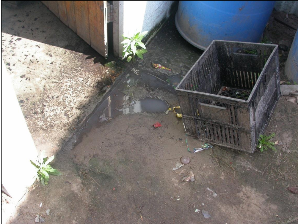
Figure 21: An example of water draining out of the toilet area and standing in the yard in Driftsands
