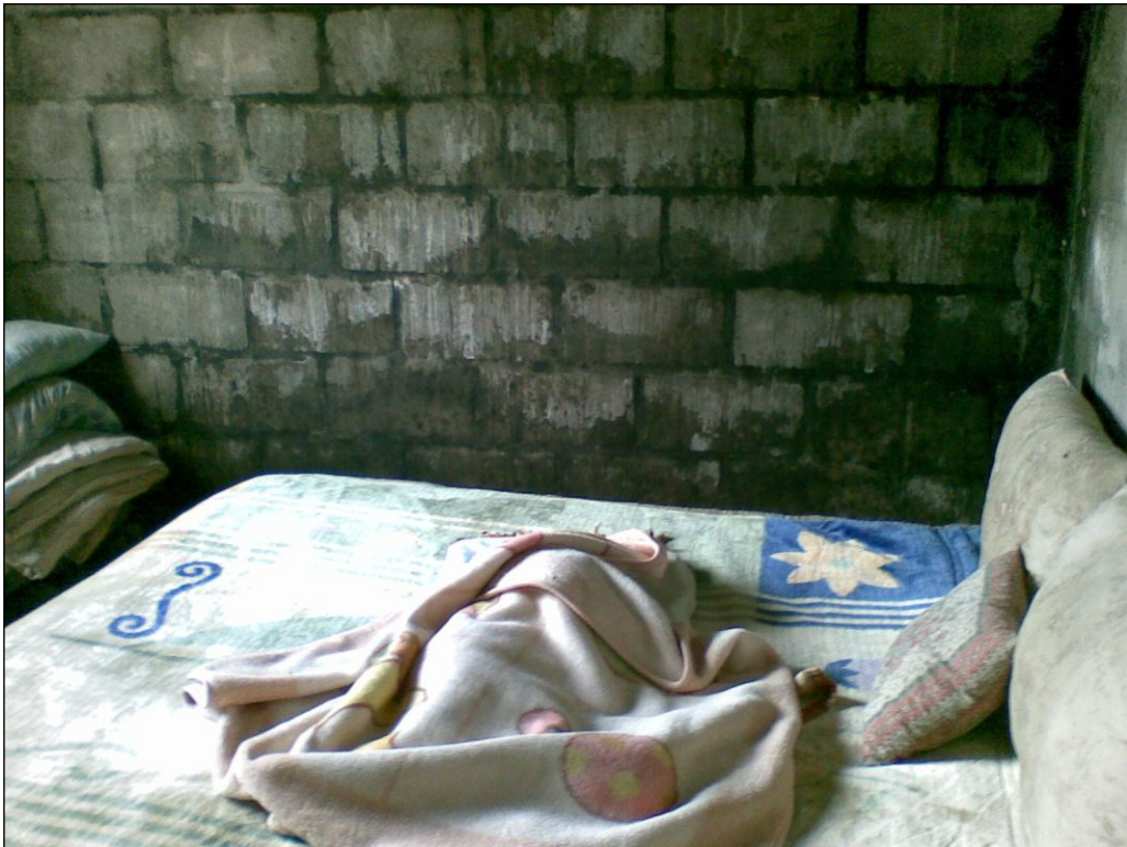
Figure 7: Dampness penetrating bedroom wall with infant sleeping on bed
